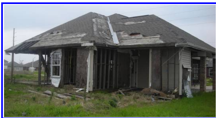
Figure 5-13. Wash-through of walls on a residential slab-on-grade structure subject to storm surge flooding from Hurricane Katrina in 2005
