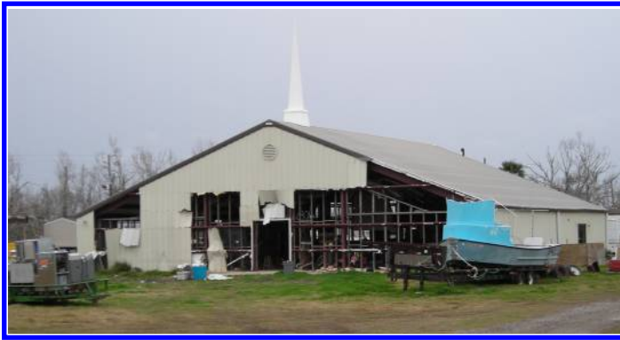
Figure 5-14. Failure of wall panels on a metal building due to storm surge flood load from Hurricane Katrina in 2005
