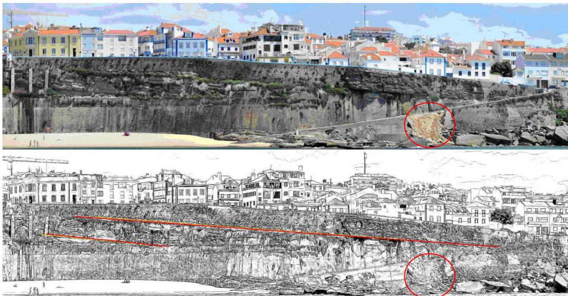
**FIG. 3. Aspect of the cliffs at Zone 3 (Fig. 2) located above and under the access road to the harbour beach (centenary retaining wall rupture highlighted by a red circle); hard carbonate layers underlined with red lines on the sketch.**
