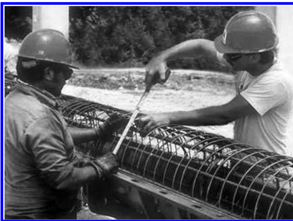
Fig. 7-2. Pole fabrication inspection
