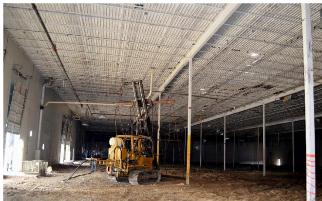
Figure 19. Equipment used to perform chemical and water injection inside the warehouse.
