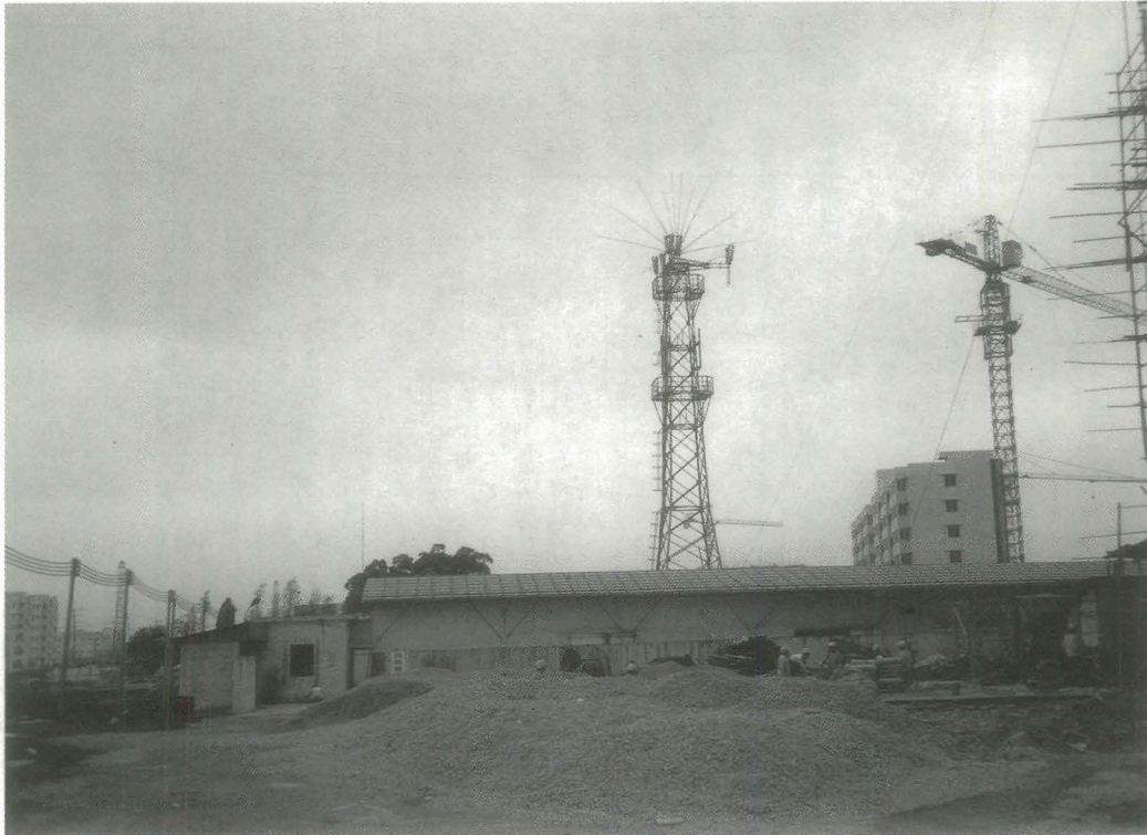
Figure 14.15 Wireless cell antenna mounted on lattice-type structure.
