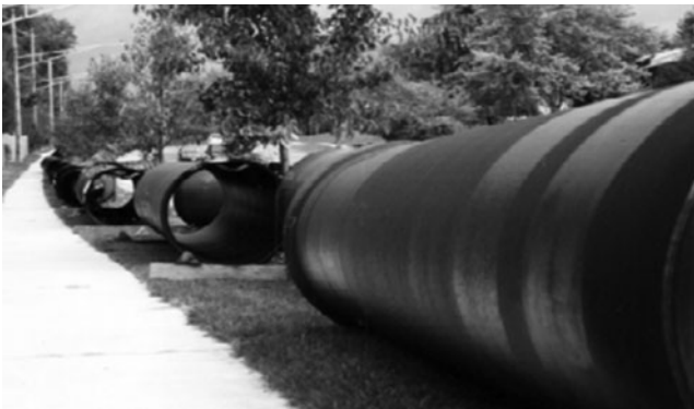
Figure 12-3. Pipe storage on the job site. Courtesy of the Watek Engineering Corporation.
