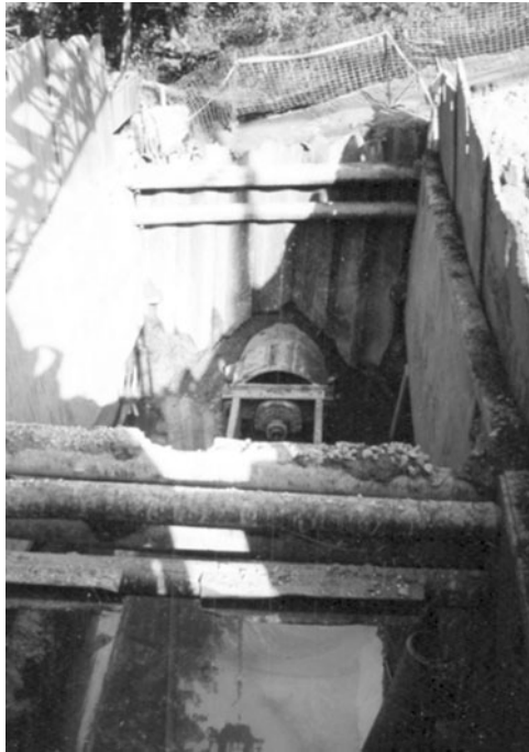
Figure 12-5. A typical pit for earth boring and pipe jacking. Courtesy of the Watek Engineering Corporation.
