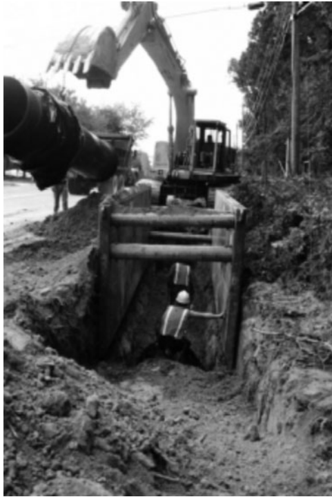
Figure 12-6. Pipe-laying activity using a trench box. Courtesy of the Watek Engineering Corporation.
