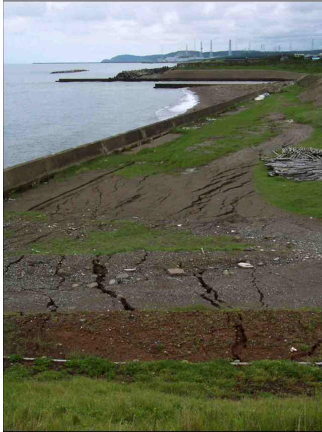
Fig. 3.186. Extensive ground failures in proximity to the seawall located near the mouth of the Sabaishi River (approximately N37.38868° E138.56413°).
