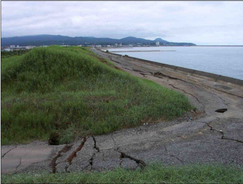
Fig. 3.189. Extensive ground deformations adjacent to the embankment and seawall.
