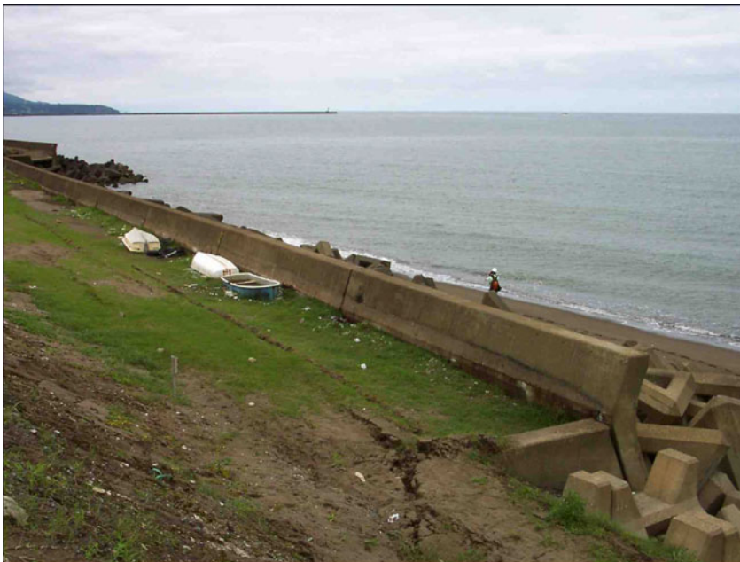
Fig. 3.182. Eastern end of the seawall located near the mouth of the Sabaishi River (approximately N37.38868° E138.56413°). Lateral spreading behind the wave armor units, as well as ground settlement and minor sea wall damage was widespread.
