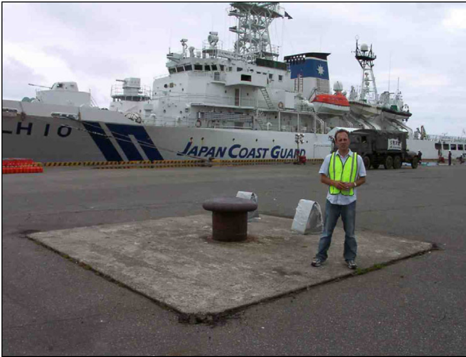
Fig. 3.174. Kashiwazaki Port—eastern berth. Evidence of minor settlement adjacent to a pile-supported (?) bollard anchorage located along the northern face of the terminal (N37.36680° E138.53825°).
