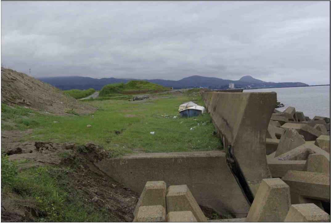
Fig. 3.183. Lateral displacement of the seawall located near the mouth of the Sabaishi River (approximately N37.38868° E138.56413°).
