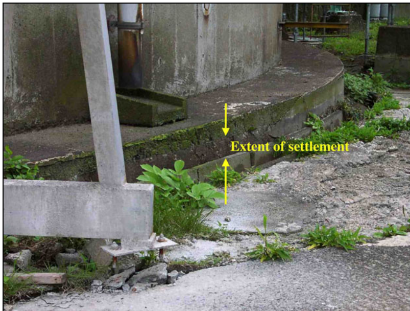
Fig. 3.179. Kashiwazaki Port (Taiheiyo Cement Facility)—Evidence of minor settlement of sandy fill adjacent to one of the large diameter tanks (approximately N37.36665° E138.53983°).
