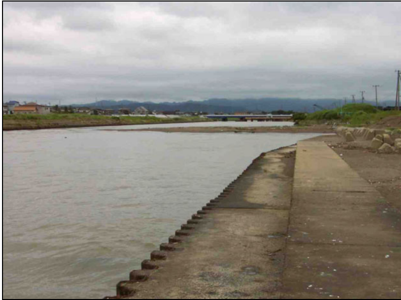
Fig. 3.181. Mouth of the Sabaishi River showing the channelization and erosion control measures (approximately N37.38868° E138.56508°). The Ansei Bridge is visible in the background.
