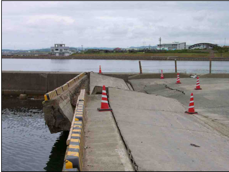
Fig. 3.178. Kashiwazaki Port—eastern berth. Significant liquefaction-related damage to the quay walls located adjacent to the U River (approximately N37.36680° E138.53825°).
