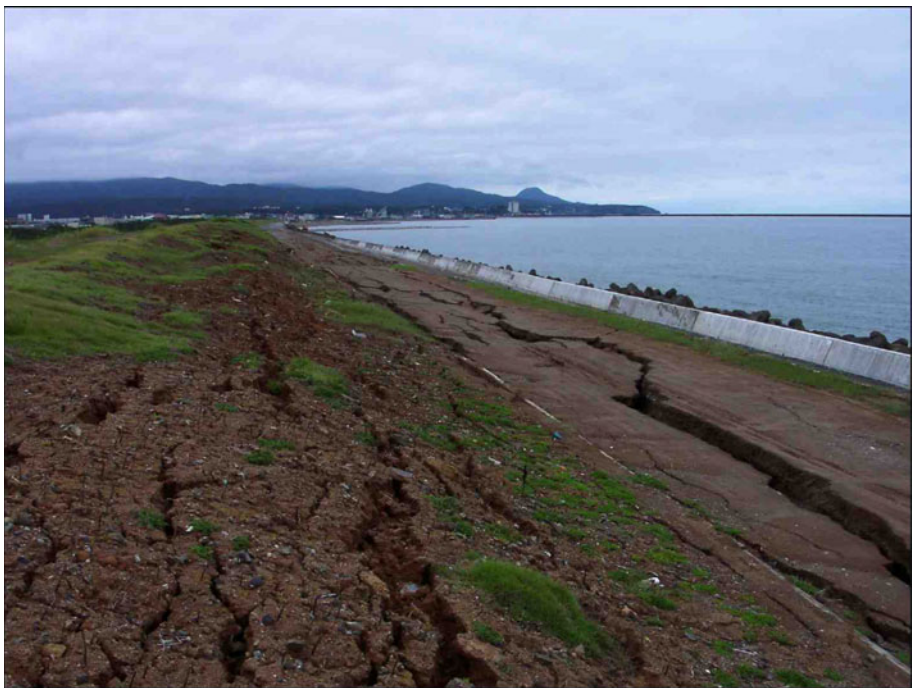
Fig. 3.188. Representative ground cracking and lateral displacement of the clayey earth embankment adjacent to the seawall.
