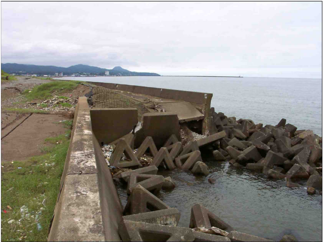
Fig. 3.184. Partial collapse of a portion of the seawall (approximately N37.38868° E138.56413°).
