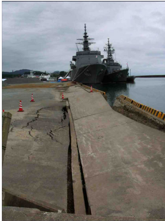
Fig. 3.177. Kashiwazaki Port—eastern berth. Significant liquefaction-related damage to the quay walls located at the eastern edge of the terminal adjacent to the mouth of the U River (approximately N37.36680^{\circ} E138.53825^{\circ} ).
