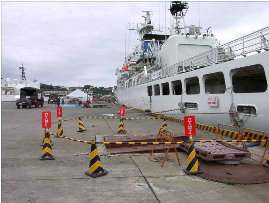
Fig. 3.175. Kashiwazaki Port—eastern berth. Evidence of very minor lateral movement of quay walls and minor settlement located along the northern face of the terminal (approximately N37.36680° E138.53825°).
