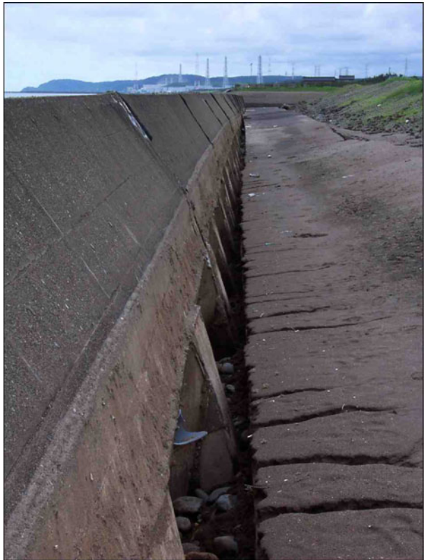
Fig. 3.187. Evidence of seawall rotation, ground settlement, and lateral spreading at the toe of the benched embankment.
