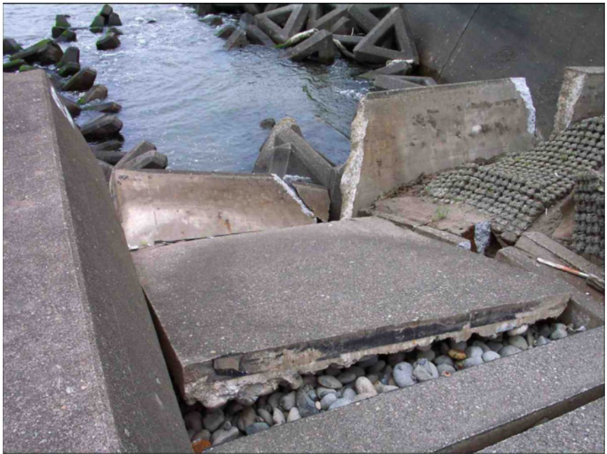
Fig. 3.185. Close-up of the collapsed portion of the seawall showing the clean cobble backfill (N37.38868° E138.56413°).
