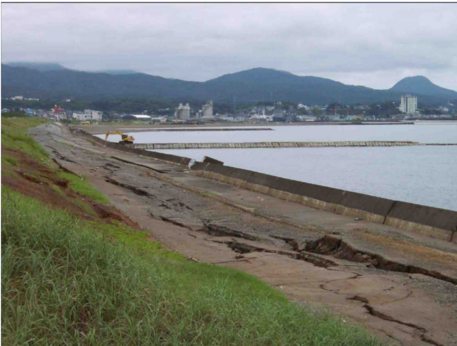
Fig. 3.190. Ground deformations adjacent to the embankment and seawall.
