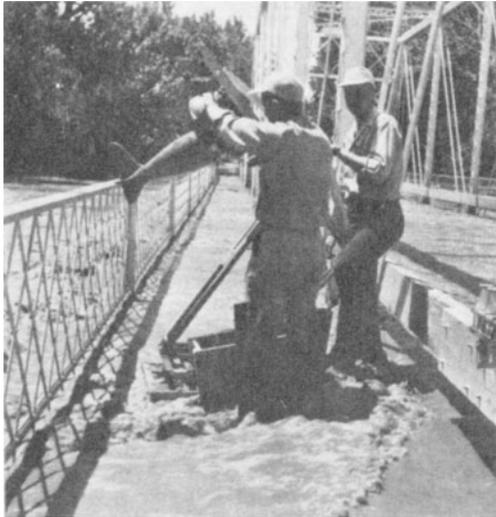
**Figure 3.21** Equipment for collection of suspended-sediment samples, Solomon River at Beloit, Kansas: US P-46 sampler and four-wheel crane (Photograph by United States Geological Survey).
