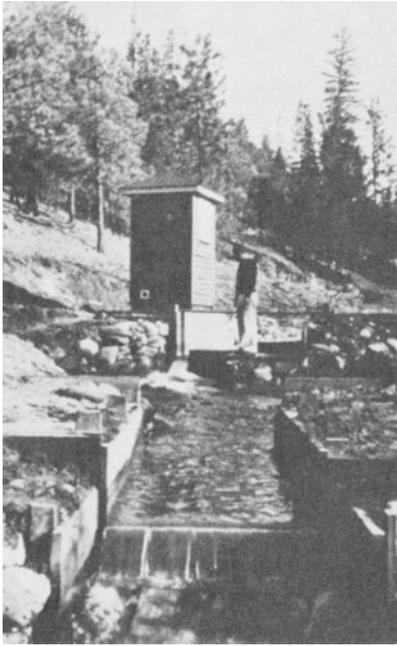
**Figure 3.24** Streamflow and sediment measuring station, Pine Creek above Barry Placer Division near Idaho City, Idaho; broad-crested weir with rectangular flume for low stages; overfall structure for sediment sampling in foreground (Photograph by United States Geological Survey).
