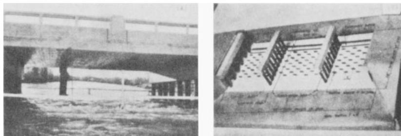
**Figure 3.23** Turbulence flume, Middle Loup River near Dunning, Neb.: (A) view looking upstream towards turbulence flume, water discharge 350 cfs; (B) skeleton model of turbulence flume (Photographs by United States Geological Survey).
