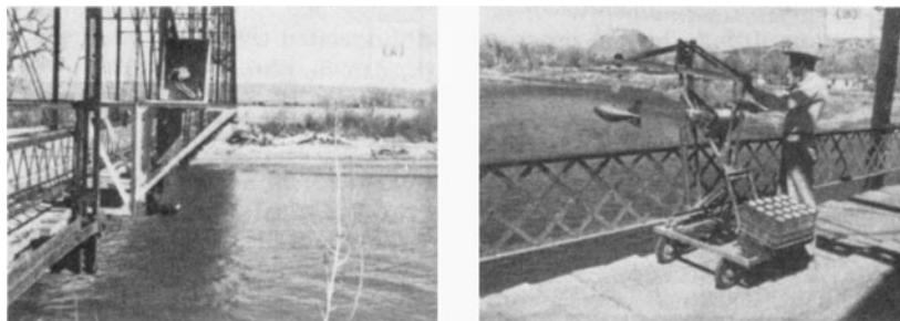
**Figure 3.20** Equipment for collection of suspended-sediment samples: (A) US D-49 sampler installation near Manderson, Wyo.; (B) US D-49 sampler and four-wheel crane near Kane, Wyo. (Photographs by United States Geological Survey).
