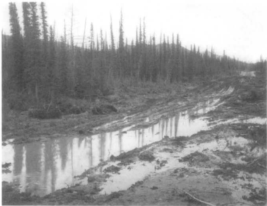
Figure 47. Road construction (2): (A) Shallow rooted trees are easily felled by bulldozer in clearing ground for road construction. The turf and top soil are also scraped, thereby exposing and allowing underlying permafrost to thaw. (B) Denuded of the insulating vegetative blanket, the melt of ground ice turns the road into an impassable quagmire (both photos courtesy of Bureau of Public Roads).
