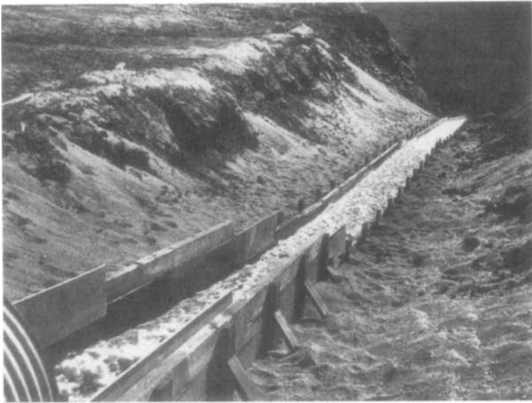
Figure 52. Two views (A, B) showing an extended spillway from a culvert on the Alaska Highway that was constructed in order to prevent road shoulders from accelerated erosion and damage (both photos by S. W. Muller).
