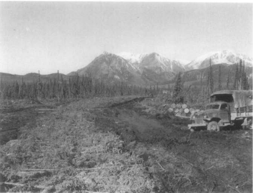
Figure 48. Road construction (3): (A) Vegetation on the path of a road is cut (not bulldozed) and spread over the ground to insulate and thus prevent the thaw of underlying permafrost. (B) Vehicular traffic at this stage of construction should be kept to a minimum (both photos courtesy of Bureau of Public Roads).
