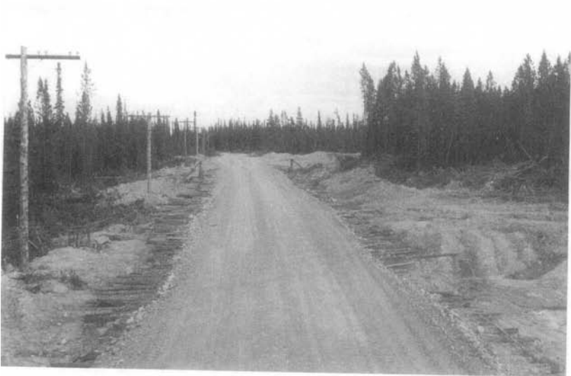
Figure 49. Road construction (4): (A) Non-frost-active basecourse aggregate (gravel) is dumped on the vegetative blanket; (B) Additional fill on shoulders insures better stability of the road. More fill should be placed on the shoulder than is shown in the picture and the material (berm) should be graded to facilitate proper functioning of snow-removing equipment (both photos courtesy of Bureau of Public Roads).
