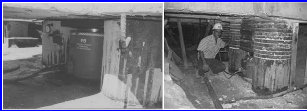
FIG 4 Jack system before and after the straightening
