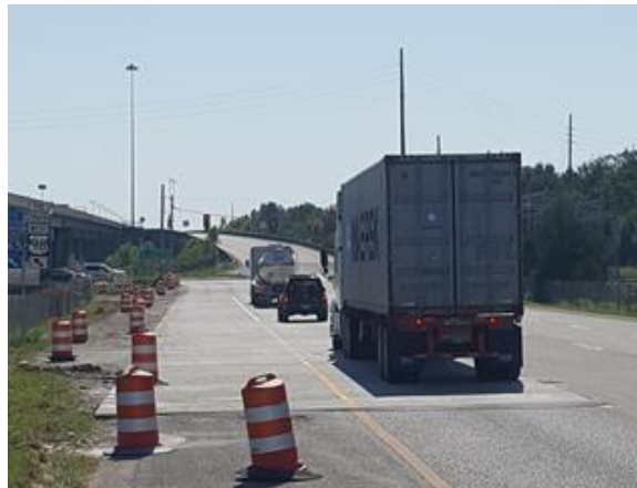
Figure 9. Completed precast pavement installation.
