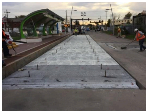
Figure 12. The north bus pad rehabilitation - panels with leveling lifts engaged.
