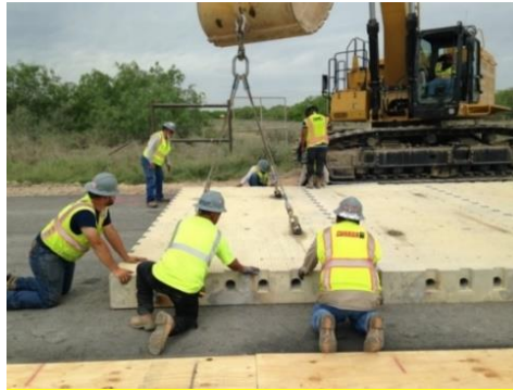
Figure 17. A panel being placed on the HMA base.
