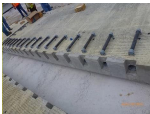
Figure 16. Typical panel with dowel bars ready to be placed in the ducts.
