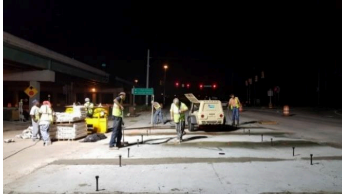
Figure 8. Using leveling bolts to set panel elevation.
