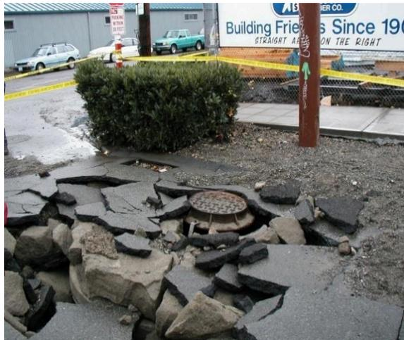
**Figure 3. Damage from a lifted top slab due to chamber pressurization.**
