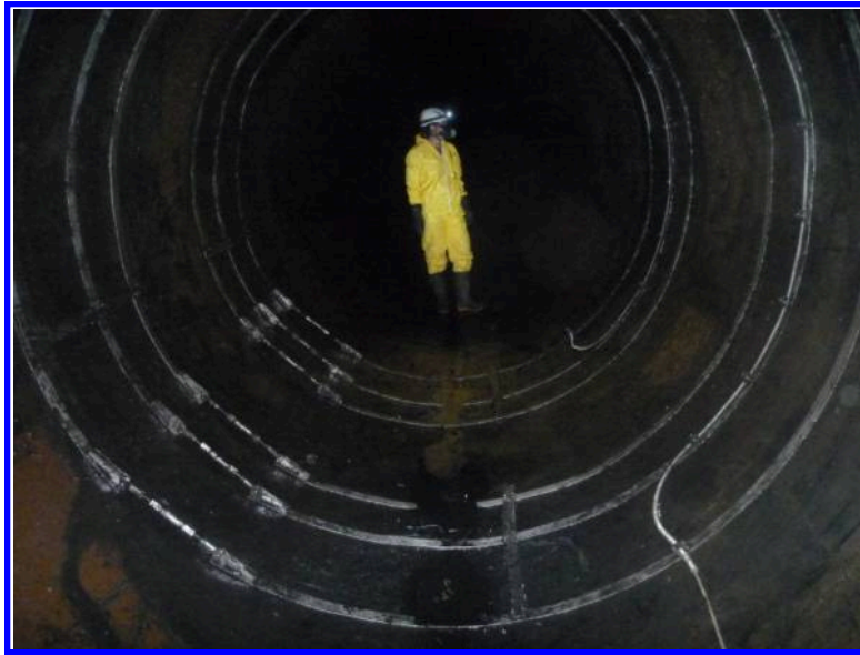
Figure 2a. Internal AFO Splice Point at MCUA
