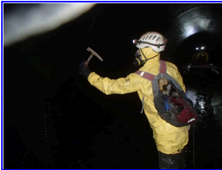
Figure 1. Inspector Sounding the 102-inch Force Main
