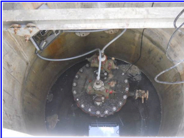
Figure 2b. External AFO Splice Point at MCUA
