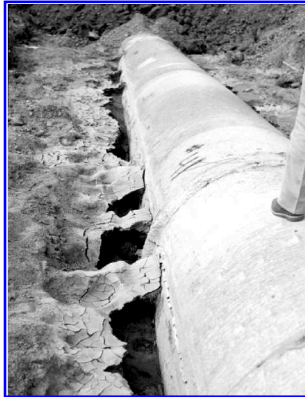
Figure 6 Too Many Fines for Saturation and Vibration
