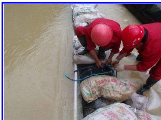
Picture 2. Silicon core pipe fastened to pipeline in rich water area
