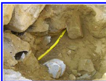
Picture 1. FOC laid in rock area
