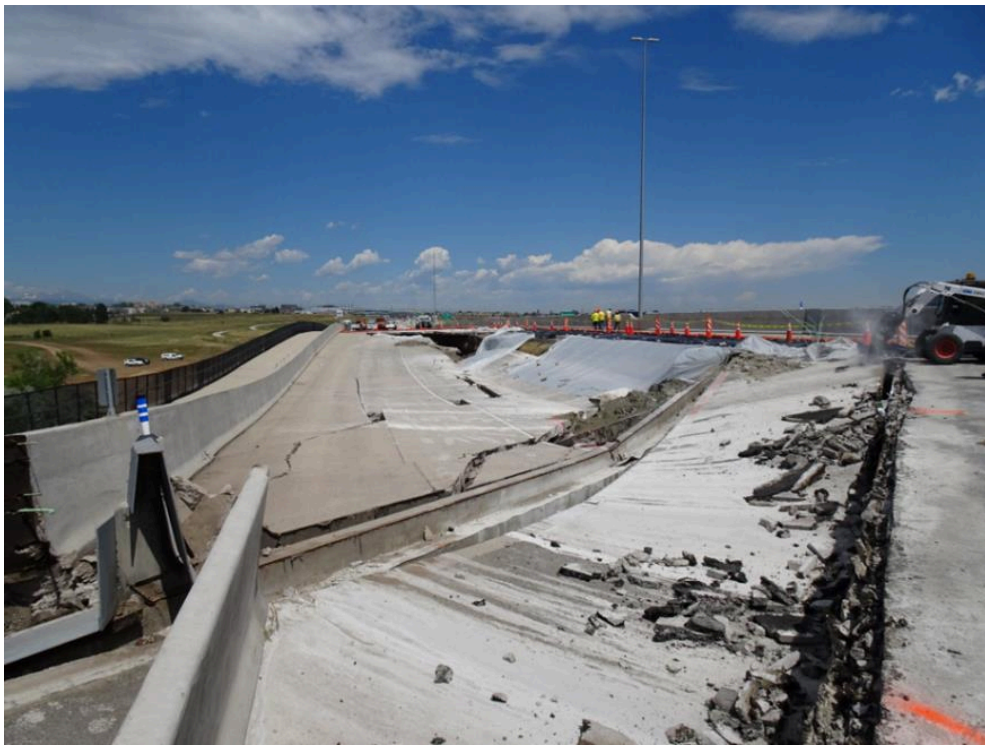
PHOTOGRAPH 2. US 36 Looking West along Eastbound Lanes on July 16, 2019 Note the lateral offset of the pedestrian guard rail barrier to the left.
