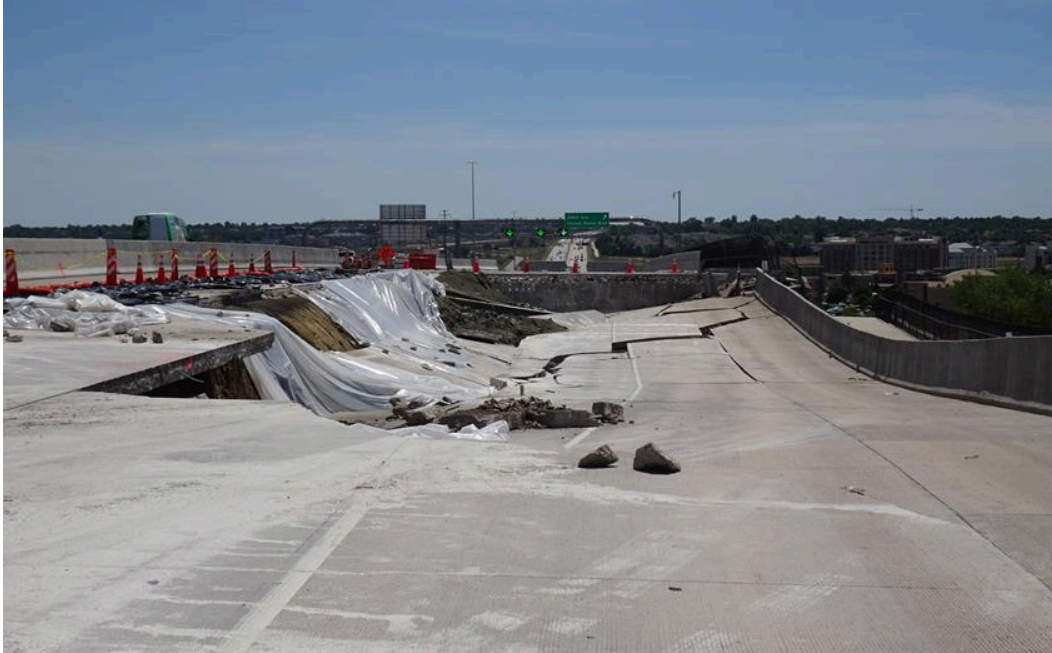
PHOTOGRAPH 1. US 36 Looking East along Eastbound Lanes on July 18, 2019 Wall supporting US 36 has dropped vertically more than 5 feet and moved laterally to the right more than 3 feet.
