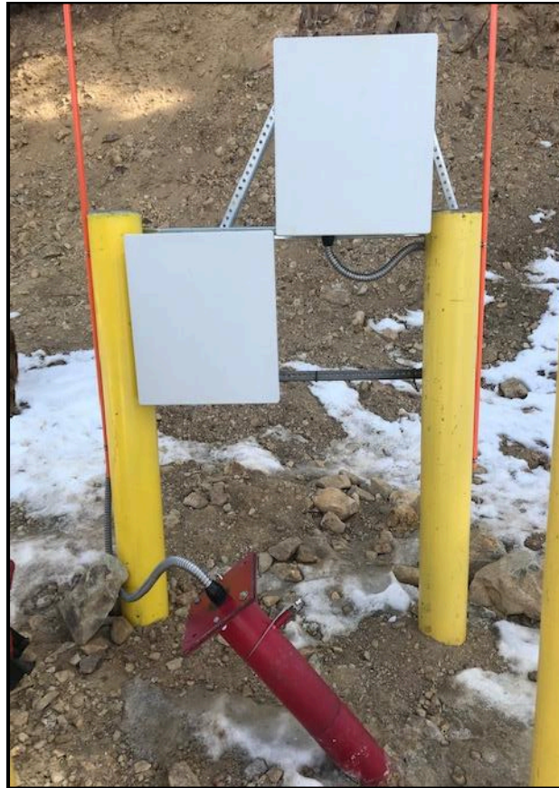
PHOTOGRAPH 1. ATPZ-2 Well Head with Protective Bollards and Instrumentation Enclosures
