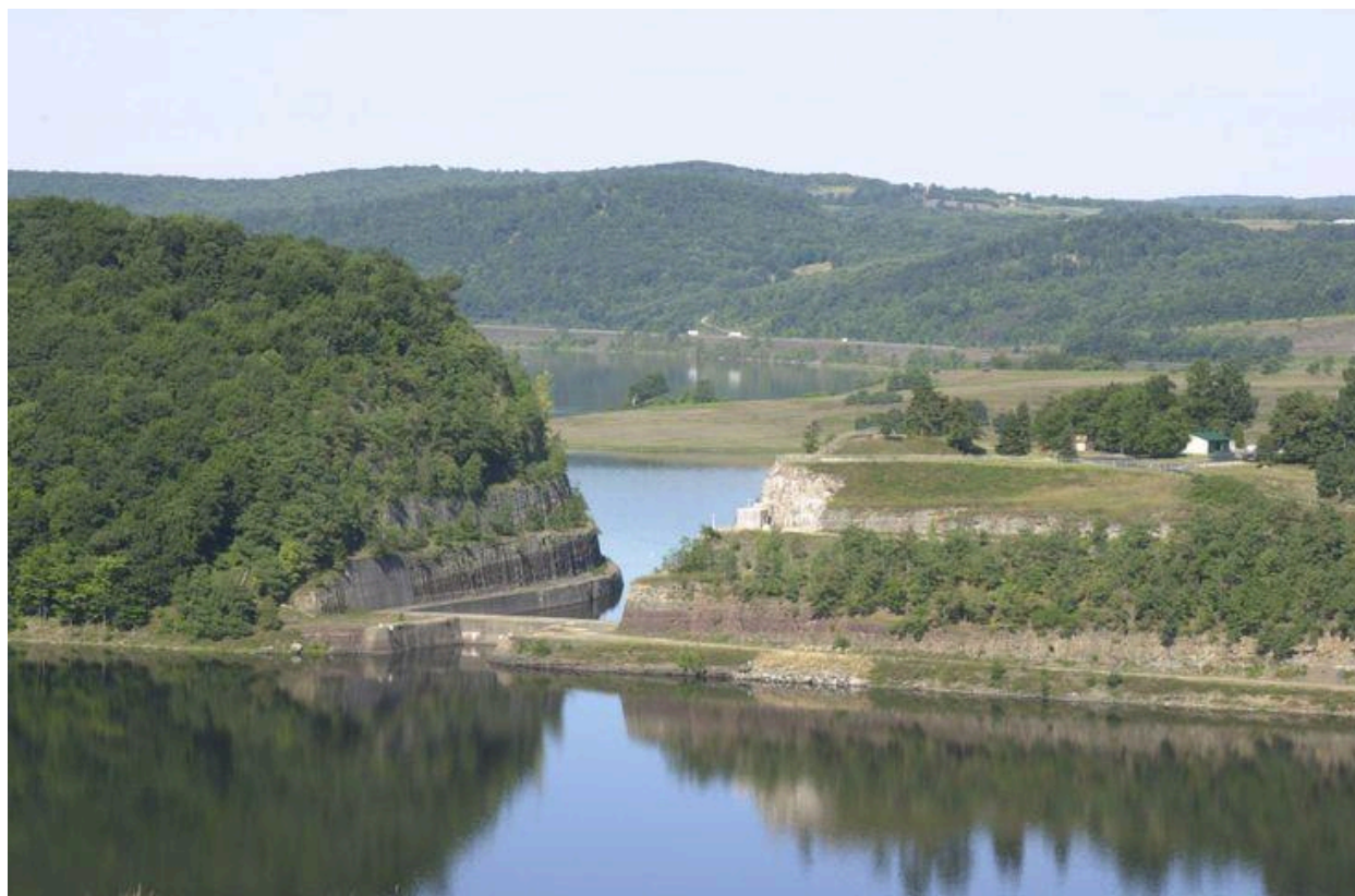
Figure 3. Connecting Channel between Hammond and Tioga, Looking from Tioga toward Hammond.
