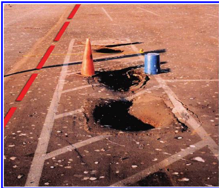
Fig. A-37. The pavement has failed entirely as a result of soil migrating from beneath the pendant wall below (indicated by the dashed line)
