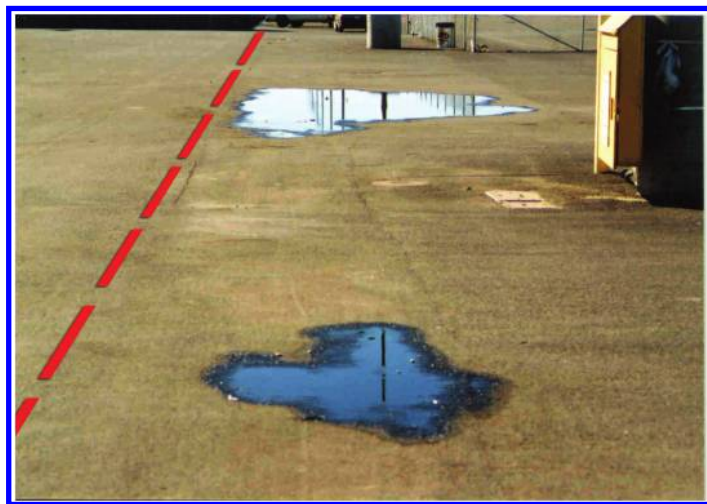
Fig. A-36. The ponding seen in this photo indicates subsidence, probably through the pendant wall below (delineated by the dashed line)
