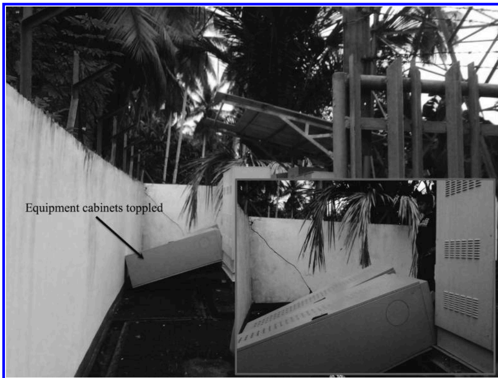
Figure 6.2. Toppled power cabinets at a BTS site outside of Padang. (Courtesy of Thomas Heriyanto)
