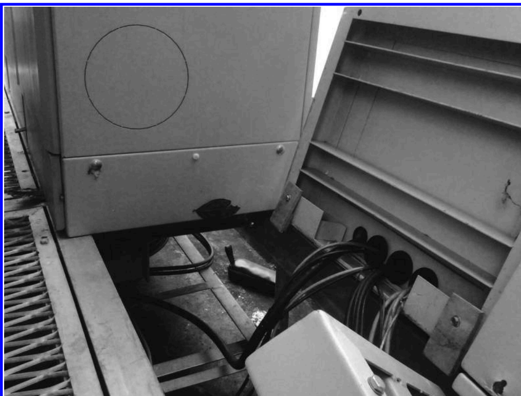
Figure 6.6. This toppled cabinet was saved by the wall. Note that there is no anchor for the equipment cabinet. (Courtesy of Thomas Heriyanto)
