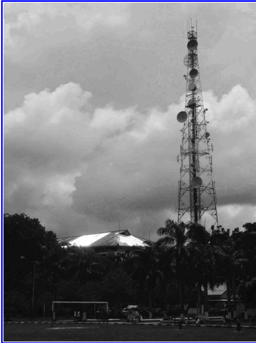
Figure 6.7. Typical standalone steel lattice tower shows good performance
