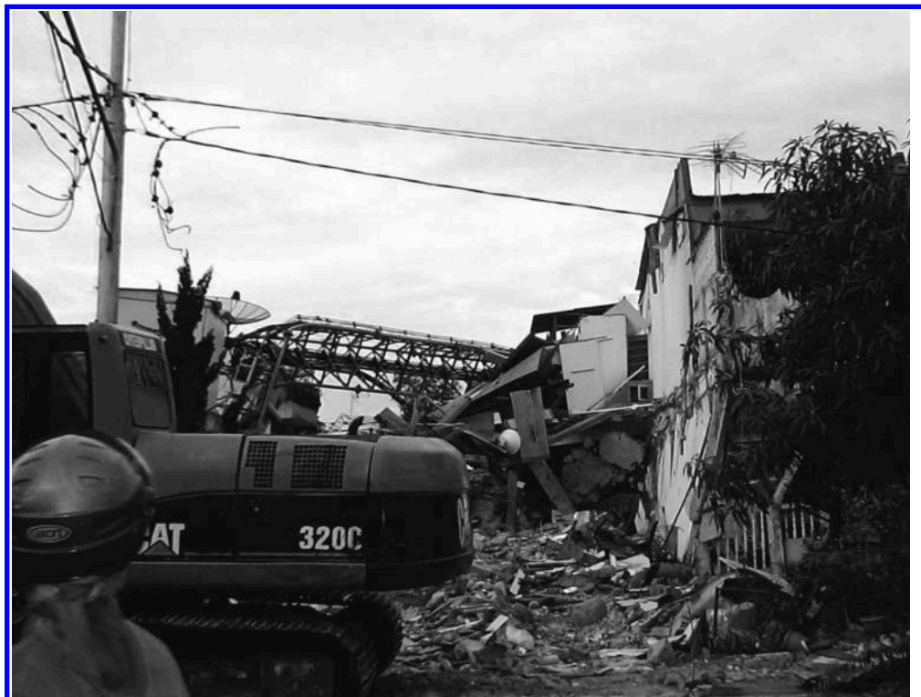
Figure 6.13. This BTS tower collapsed when the buildings around it collapsed in the earthquake. (Courtesy of Fire Department, Padang)
