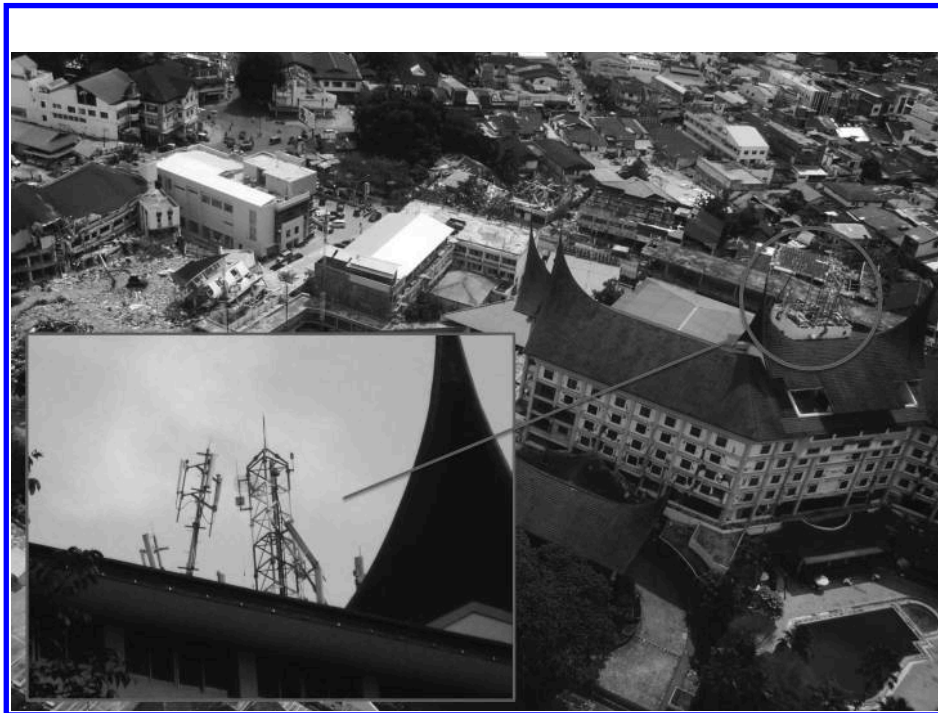
Figure 6.8. Roof-top mounted BTS antenna poles failed when the building failed. There were three service providers located on the roof of this 5-star hotel in Padang.
