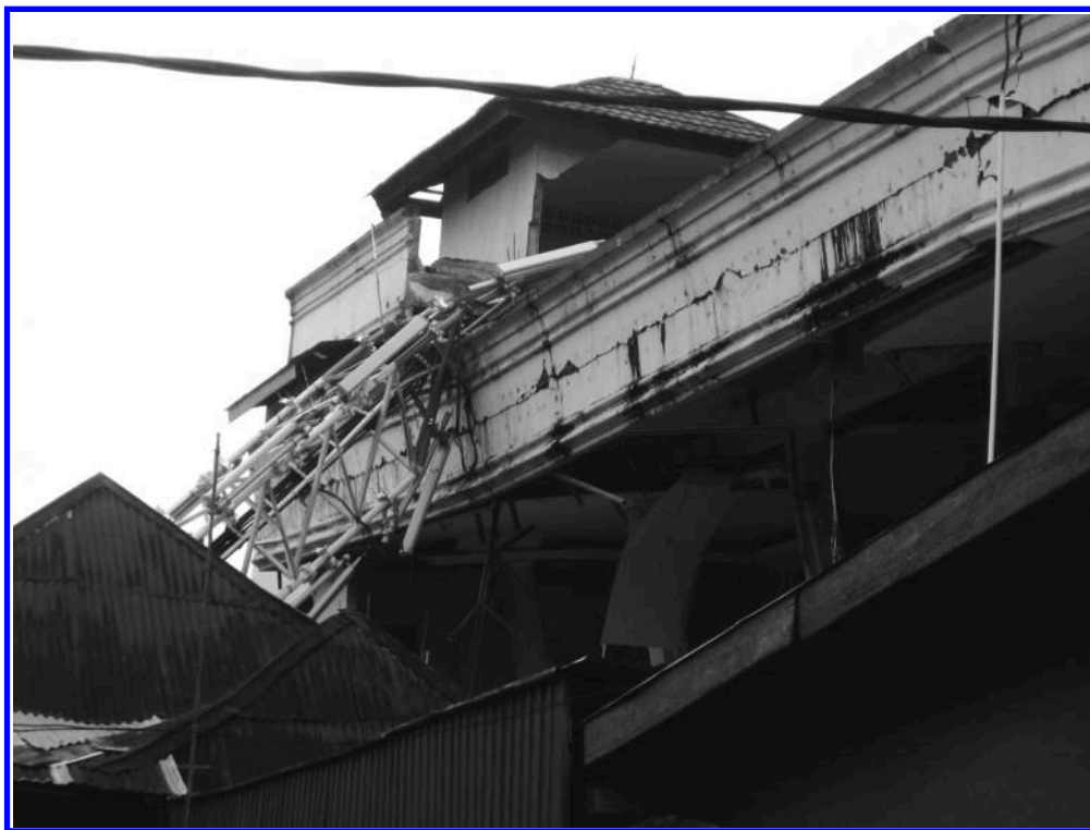
Figure 6.11. Detail view of the collapsed tower and antennas (Courtesy of Thomas Heriyanto)
