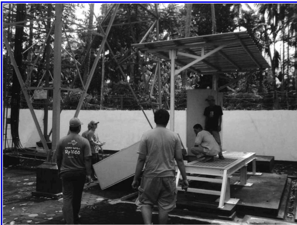
Figure 6.4. One of the two cabinets toppled at this BTS (Courtesy of Thomas Heriyanto)
