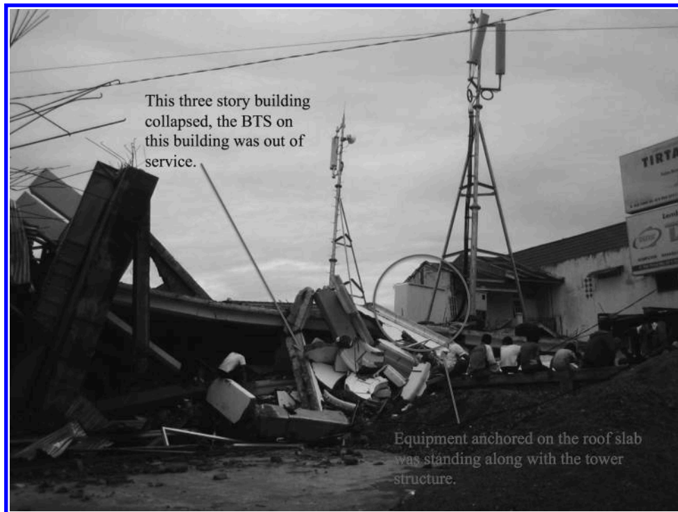
Figure 6.12. The tower and the equipment housing do not look damaged, but power was cut off when the building collapsed. (Courtesy of Thomas Heriyanto)
