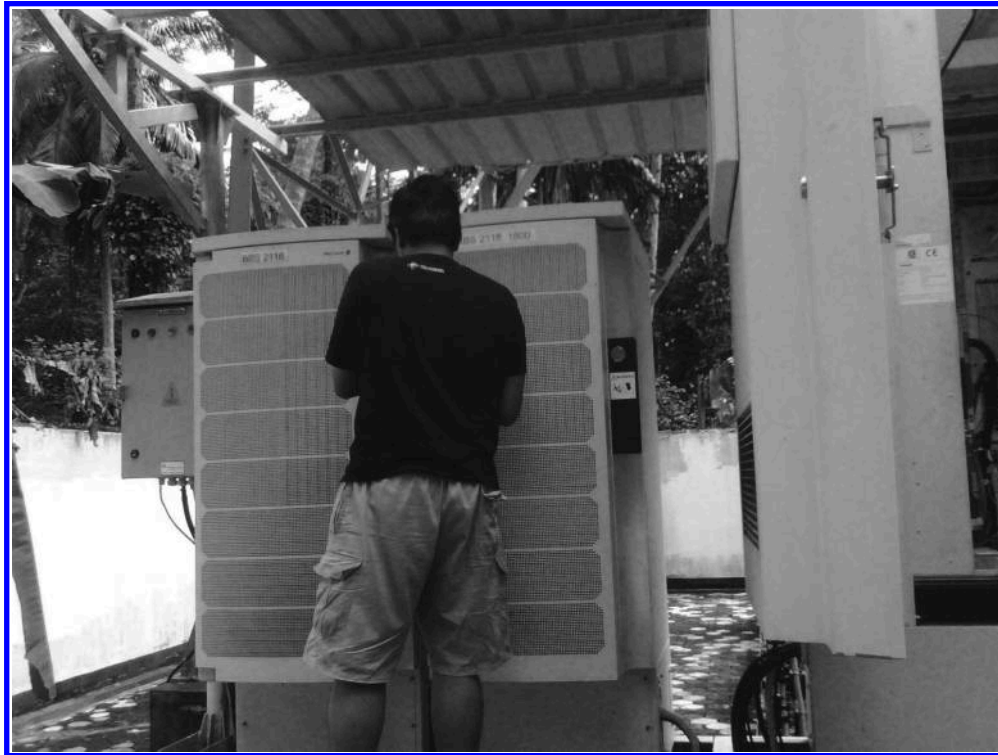
Figure 6.1. BTS with a self-contained unit, no building is required. The base is still enclosed with a wall for security. (Courtesy of Thomas Heriyanto)
