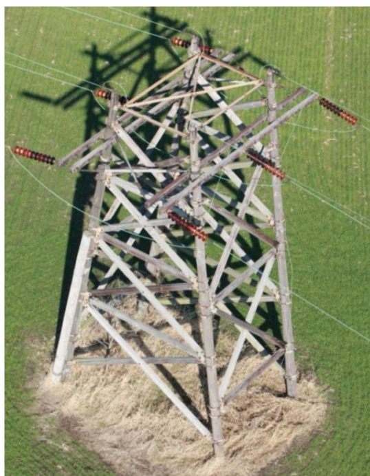
Figure 6 – Wood Lattice Structure Photo Courtesy of Ameren Illinois
