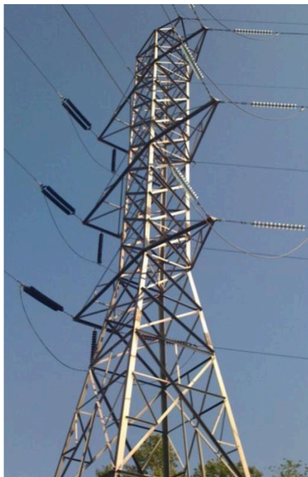
Figure 5 – Aluminum Lattice Tower Photo Courtesy of Exelon
