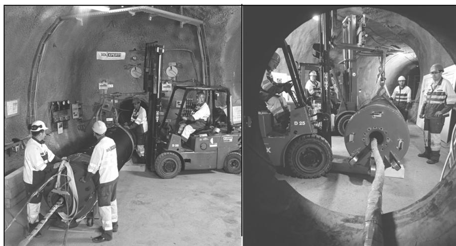
Figure 12: Megapacker before the emplacement into the microtunnel. Cables and lines pass through the megapacker centre pipe; source: COMET Photoshopping GmbH.
