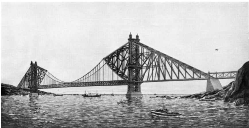
Figure 4-18. Strauss's original plan for the Golden Gate Bridge, a hybrid structure consisting of a cantilever truss and suspension bridge.
