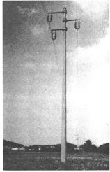
elastic and could carry significantly higher loads without cracking. The combination of prestressing technologies and spinning technologies during the mid 1950's provided a significant catalyst in the acceptance of spun concrete poles for use by electric Utilities in Europe. These prestressed, spun concrete poles were stronger, more durable, and much lighter in weight than previous types of concrete poles. The improved characteristics made these new poles easier to transport and erect.
