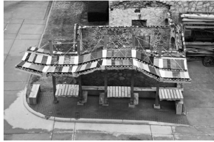
Figure 4- Final constructed pallet canopy
