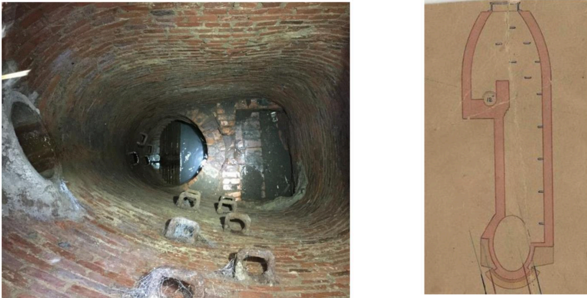
Figure 2 Irregular brick manhole with parallel 12" collector at a higher elevation
