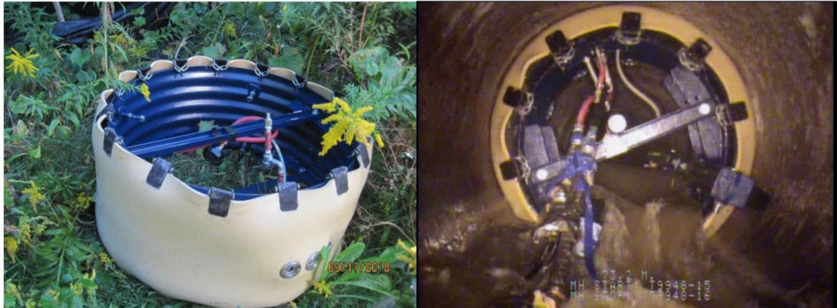
Figure 2: Inflatable grout packer before (left) and in service (right)
