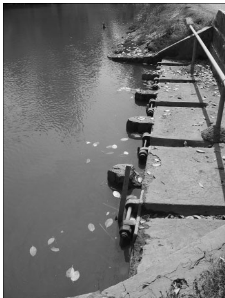
Figure 5.4.7.1. Damaged sluice gates under Andaman Island Trunk Road. (Photo by ASCE/TCLEE/EIC team.)
