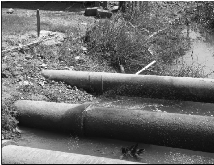
Figure 5.4.6.1. Water main leaking along South Andaman Island Trunk Road. (Photo by ASCE/TCLEE/EIC team.)
