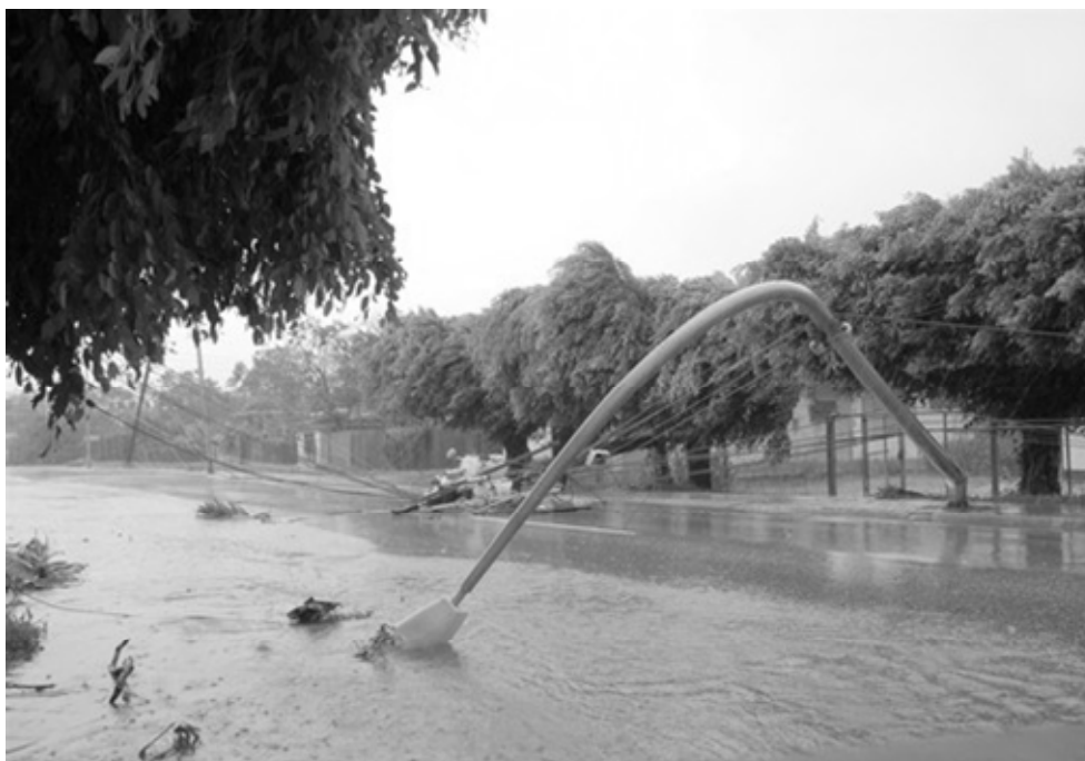
Fig. 6.2. Example of damage to cable infrastructure (Source: FEMA 543, Design Guide for Improving Critical Facility Safety from Flooding and High Winds: Providing Protection to People and Buildings, 2007.)
