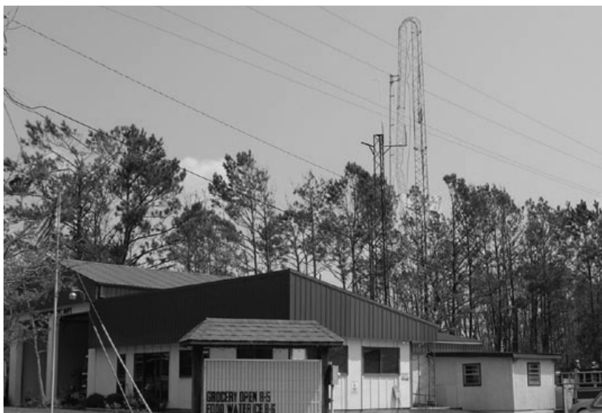
Fig. 6.1. Example of buckled antenna tower at Mississippi fire station (Source: FEMA 543, Design Guide for Improving Critical Facility Safety from Flooding and High Winds: Providing Protection to People and Buildings, 2007.)
