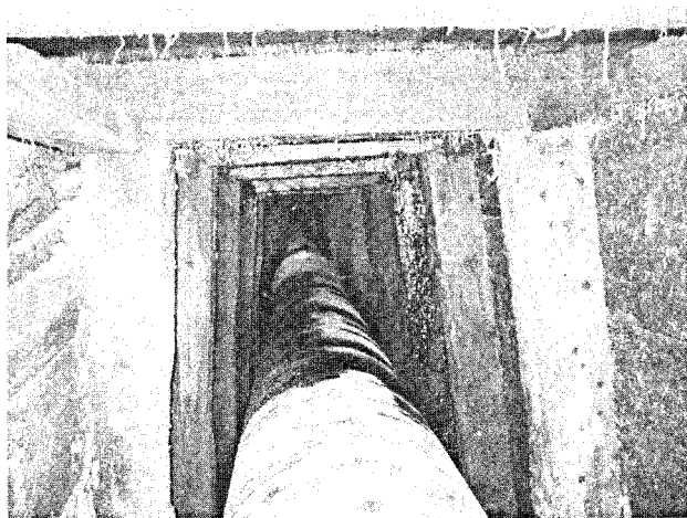
Figure 1. Timber Support in Shear Zone.
