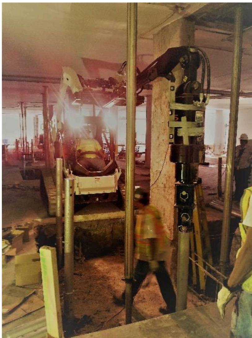
Figure 22 – Installation of helical pile
