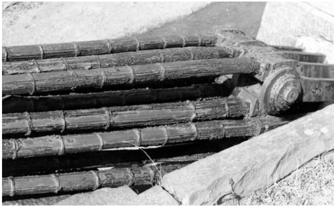
Delaware Aqueduct Anchorage. The anchorages of the Delaware River Aqueduct are still in place after 160 years of service. Although they were previously exposed to view for many years, reconstruction of a replica has caused them to be covered.
