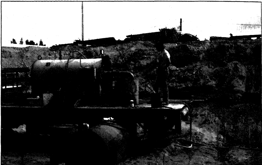
Photo 1: Steam boiler on truck, connected to thaw probes. (All photos in this series were provided by Steve Adamczak, Shannon and Wilson Consultants, Fairbanks.)
