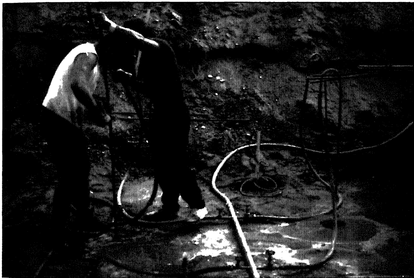
Photo 3: Inserting thaw pipes while steaming holes
