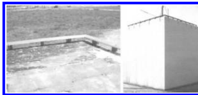
Fig. 4.8: Roof-corner vortex formation and roof-edge flow separation may be controlled by roof-edge spoilers. The diminished roof pressures are substantially smaller.
