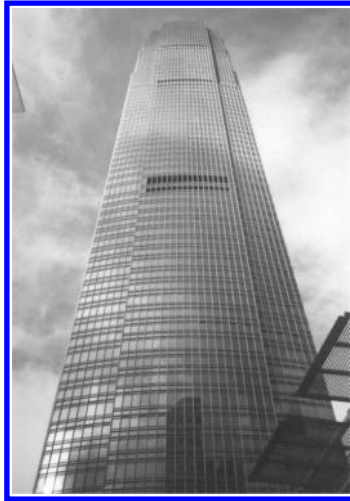
Fig. 4.7: Tall buildings resist the wind by architectural shape and structural system – Two International Finance Centre, or 2IFC, (420 m) in Hong Kong, China.
