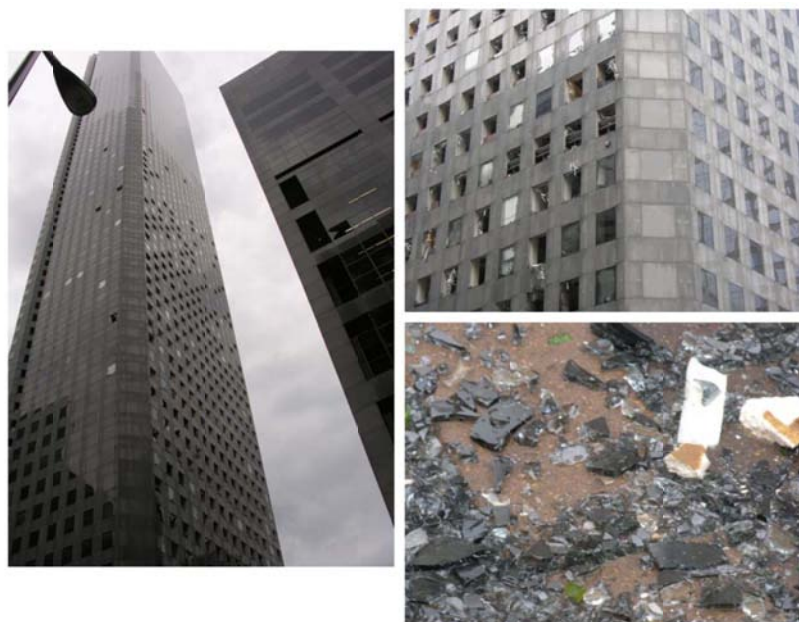
Figure 3. Damage to the JPMCT from Hurricane Ike (2008).
