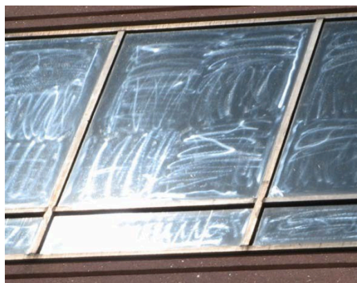
Figure 9. Unacceptable cleaning pattern remains after improper polishing operation. (RCI 2010, with permission from RCI, Inc.).
