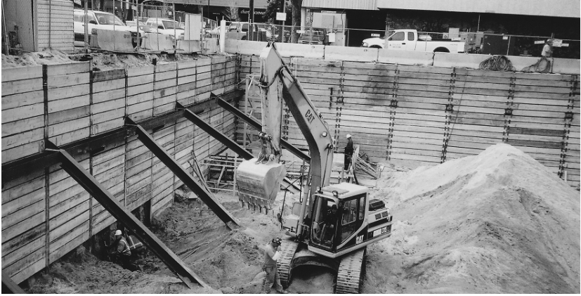
FIG. 1. Internal bracing and wale, left wall. Tiebacks, right wall, Denver, CO
