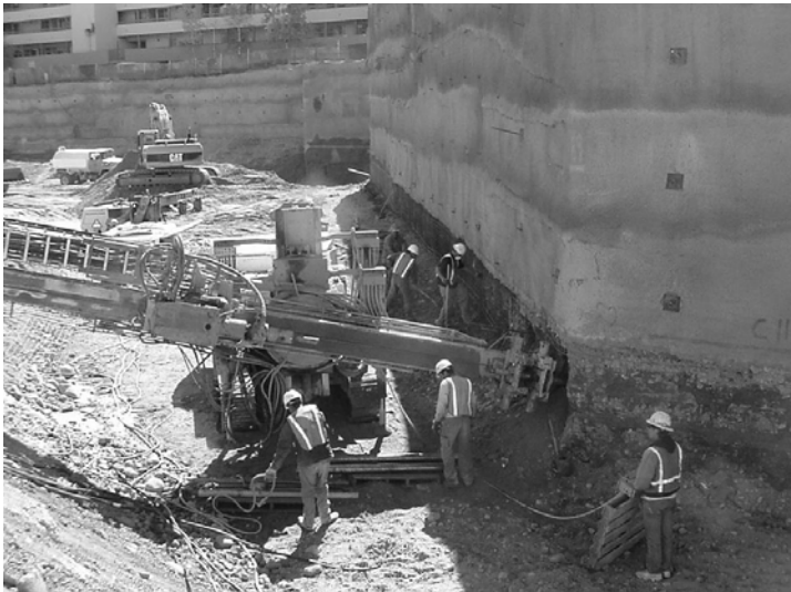
FIG. 6. Drilling Bottom Row of Soil Nails
