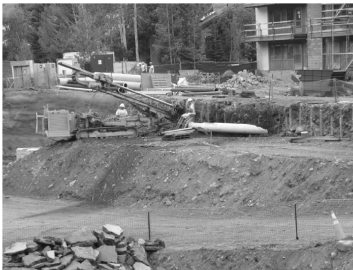
FIG. 4. Installation of the Top Row of Soil Nails
