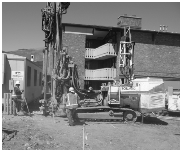
FIG. 2. Drilling Grout Columns for Soil Nail Earth Retention
