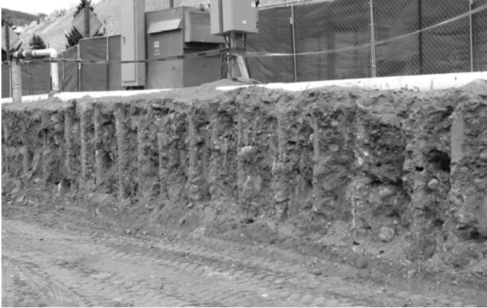
FIG. 3. Initial Excavation and Exposed Grout Columns
