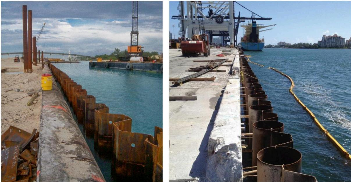
**Figure 2: Sheet Pile Wall and Combi-Wall (photos provided by Nucor-Skyline)**
