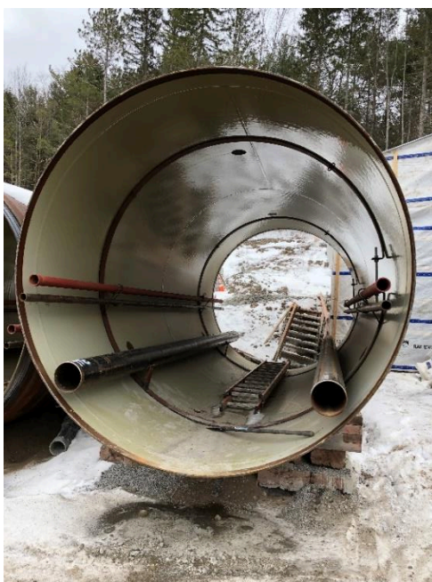
Figure 10. Polyurethane Lining
