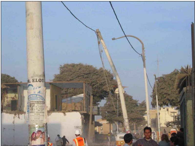
Fig. 7.25. Utility pole damaged in the street next to Hotel Candelobra, Pisco.
