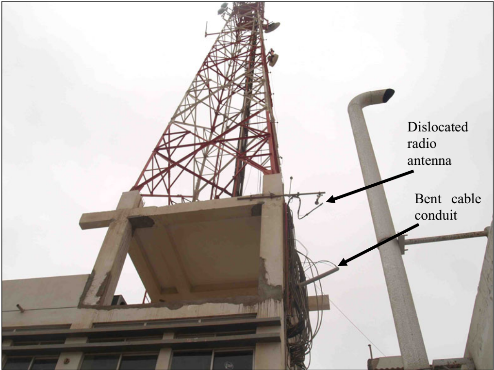
Fig. 7.19. Damage viewed from the bottom of the structure in the yard of the CO facility
