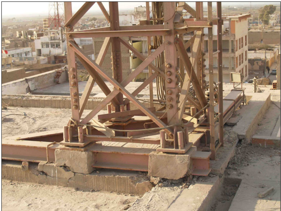
Fig. 7.26. The damage at the base of the tower
