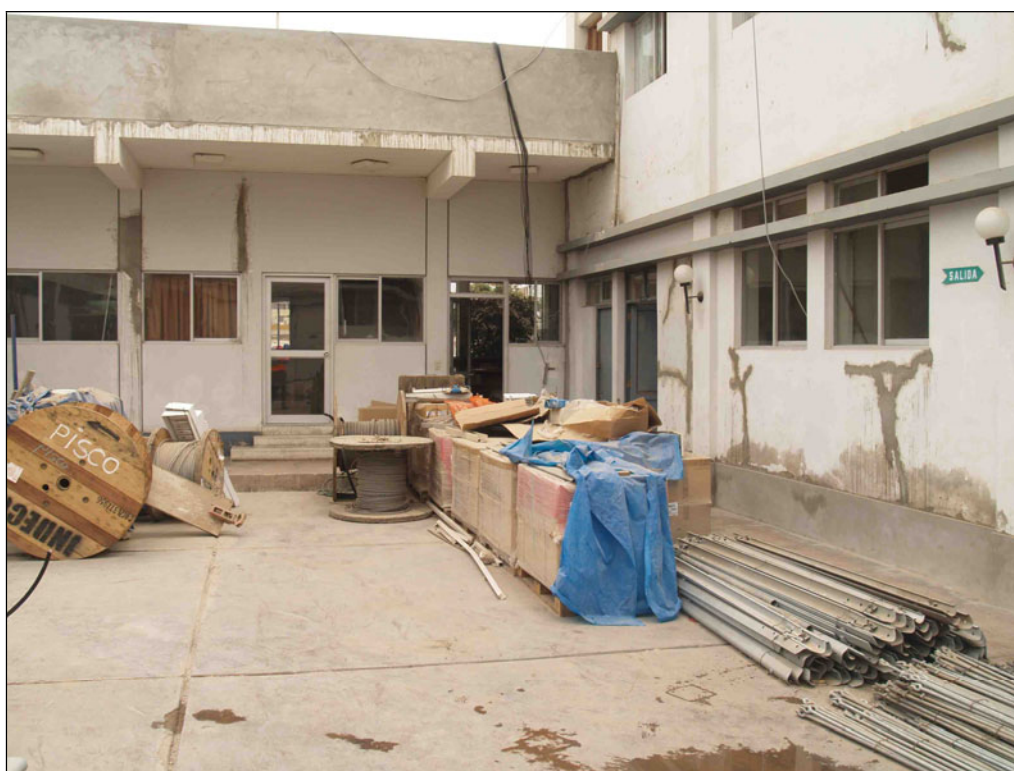
Fig. 7.21. Material for repairing damage in the yard of this CO. Note the repaired cracks on the walls.
