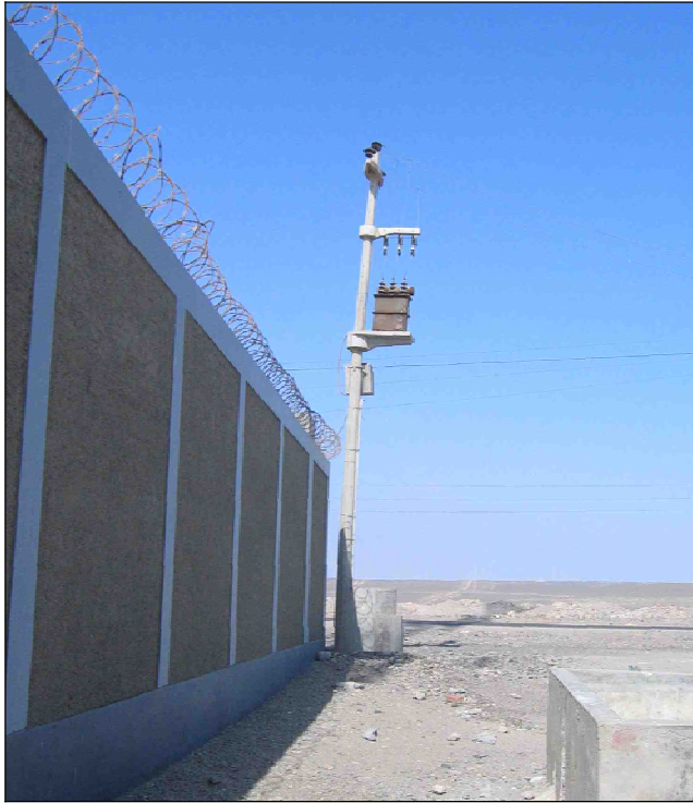
Fig. 7.32. Electric power supply to all three cell sites comes from this pole. This is an underground feed to the sites.
