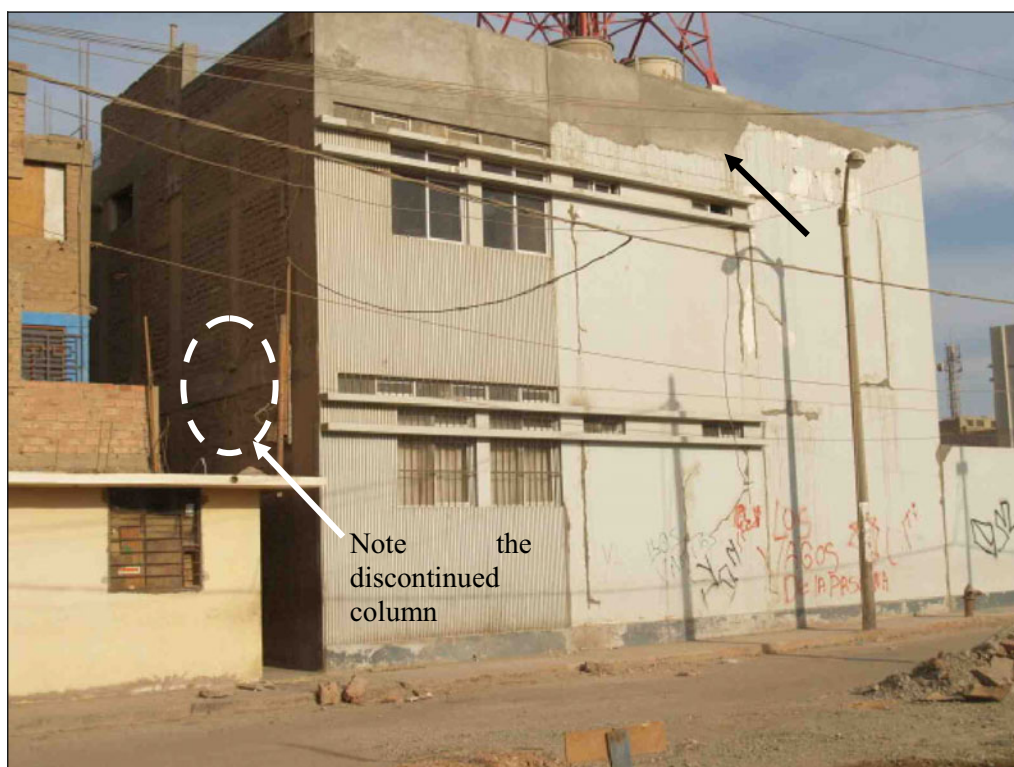
Fig. 7.20. Repaired top of the building at the back of the Telefónica CO
