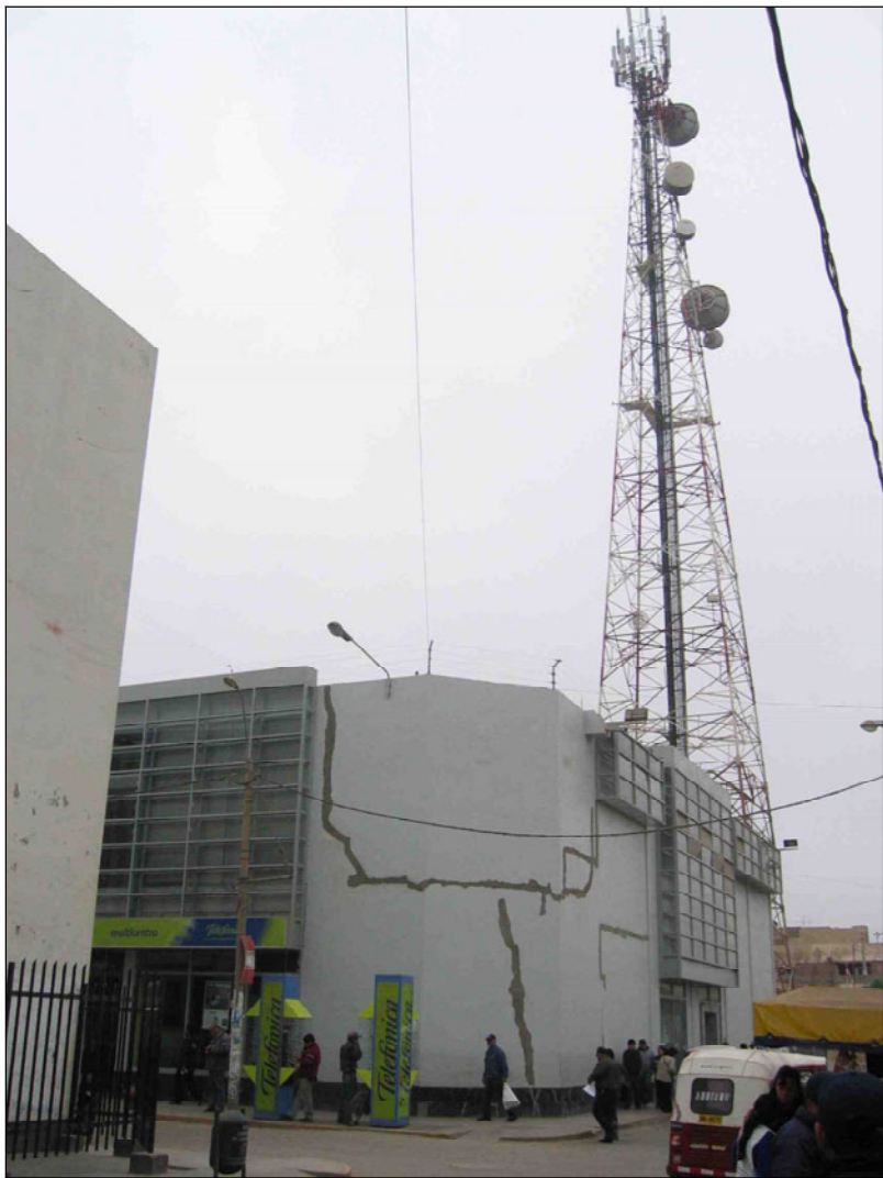
Fig. 7.28. Telefónica central office in Ica City. Surface cracks on the outside wall were fixed.
