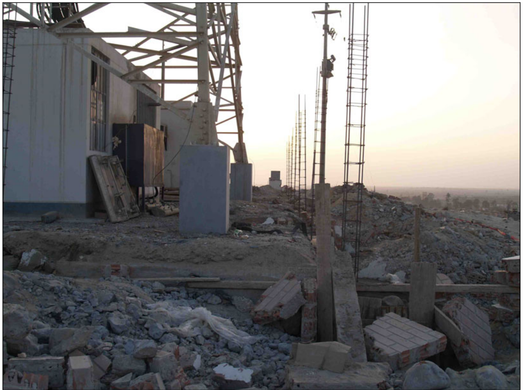
Fig. 7.34. Preparation for rebuilding the enclosure wall. Note the utility pole with a pole mount transformer serving this site.
