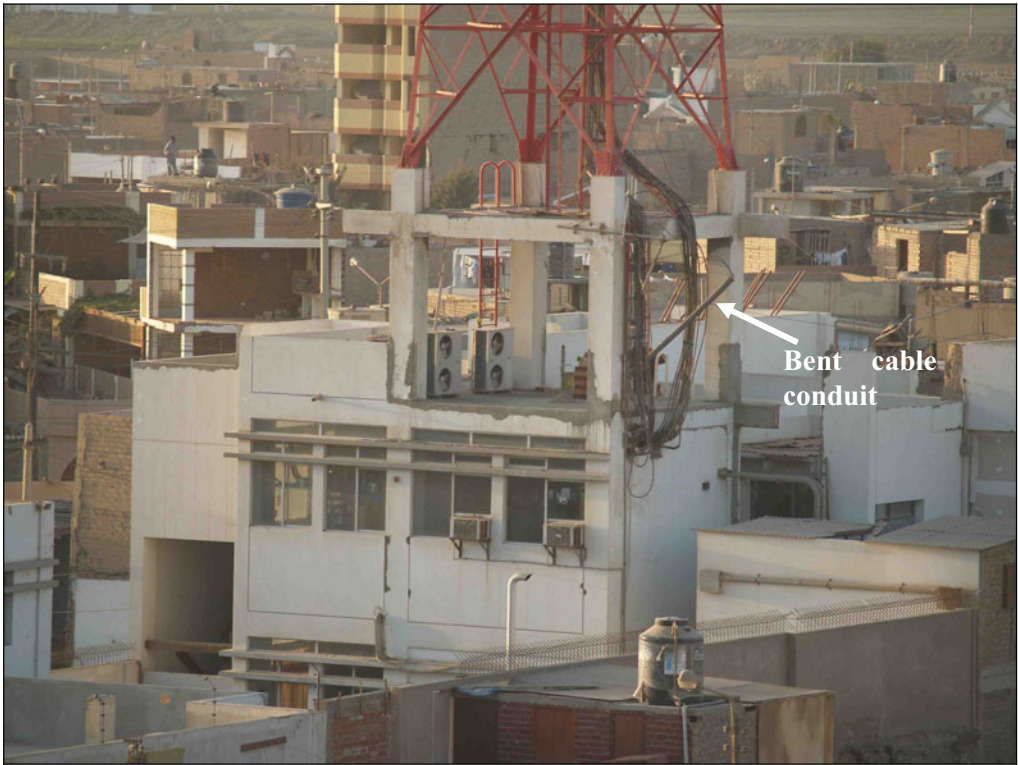
Fig. 7.18. Damage at the base of the tower support structure was repaired. Note the massive waveguide that drooped down below the tower support structure
