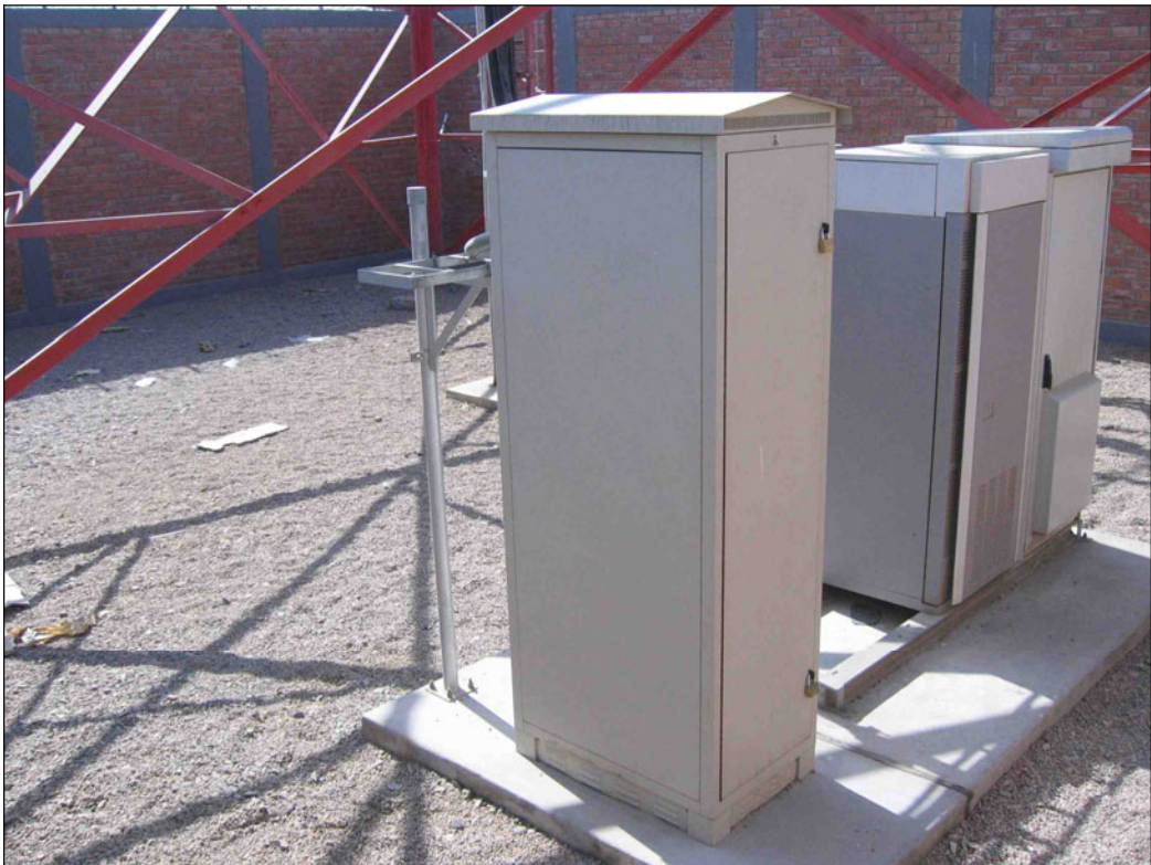
Fig. 7.31. Cell site equipment anchored on concrete pads
