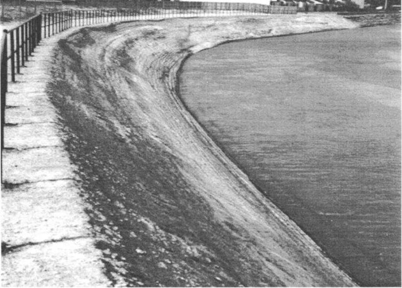
FIG. 5. Smooth trimmed soil-cement bank protection, Rillito River at Tucson, Arizona.
