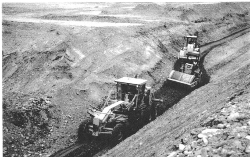
FIG. 4. Steel wheel vibratory rollers compact soil-cement along Salt River at Phoenix, Arizona.
