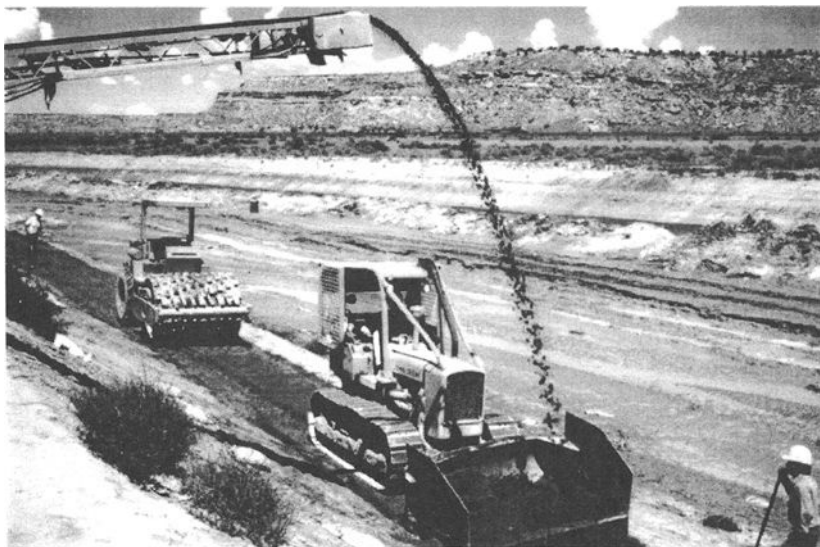
FIG. 3. Conveyor belt feeds soil-cement to spreader box, Rio Puerco, Gallup, New Mexico.
