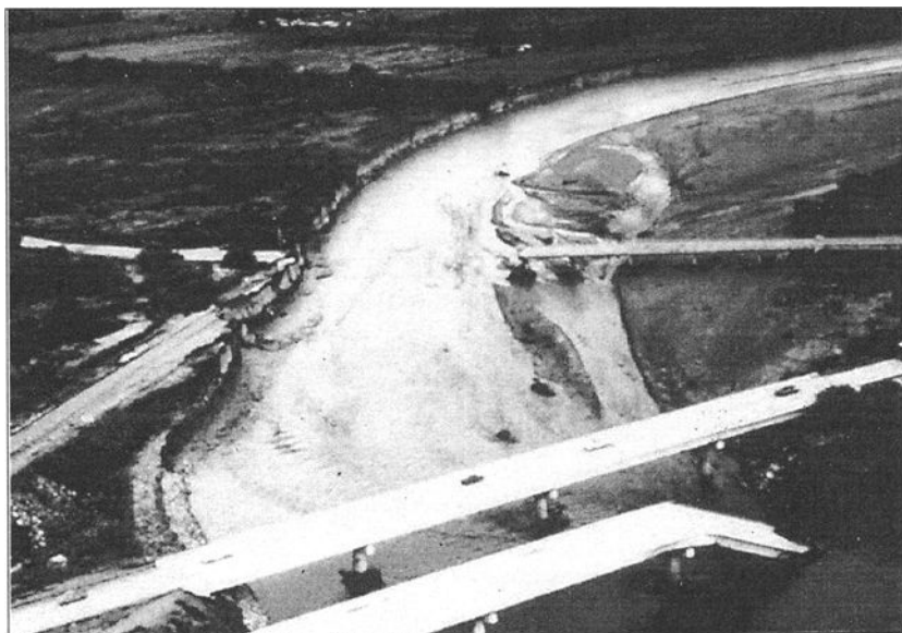
FIG. 1. Eroded sand banks and damaged bridges on the Santa Cruz River south of Tucson, Arizona.
