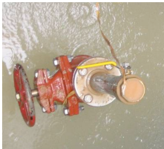
Figure 3. Mule-tape was installed in the pipeline at Insertion Point TT#2. It exits the valve and riser for connection to the Sahara sensor head.
