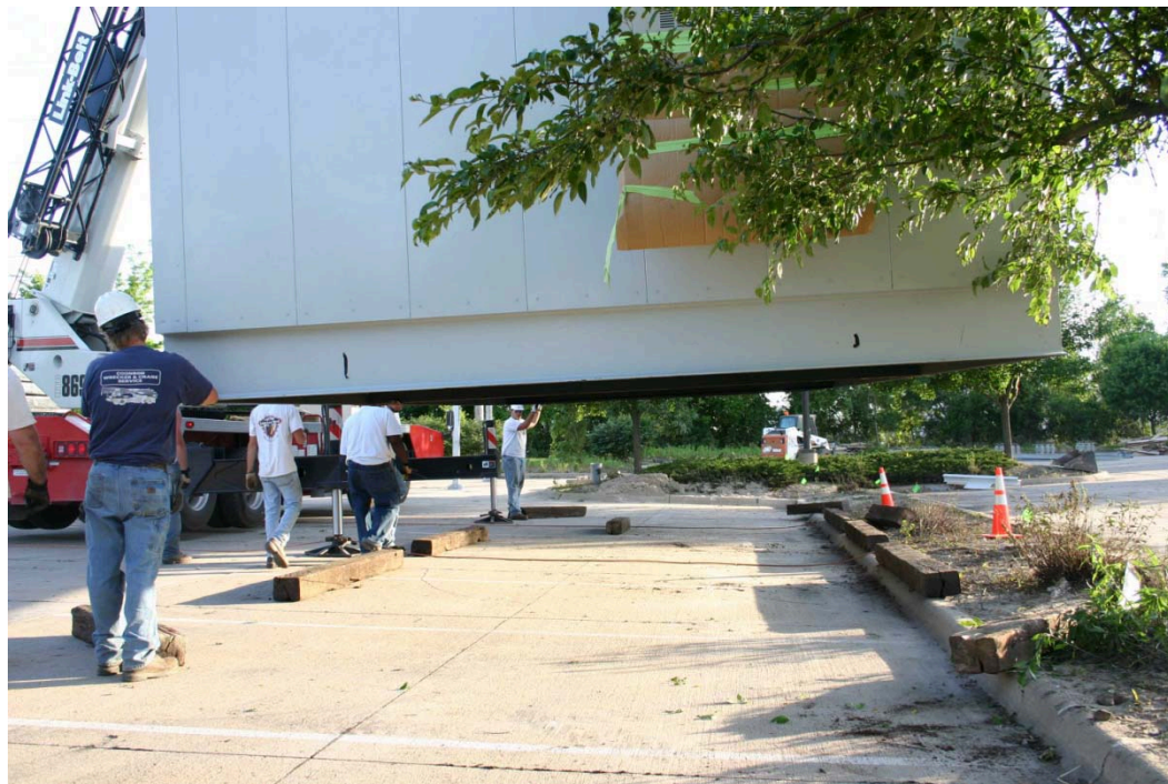
Figure 3 - Setting the 15kV Switchgear on Railroad Ties
