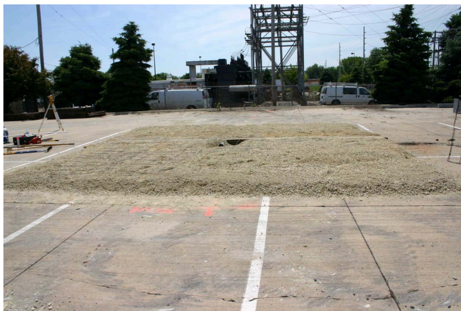
Figure 2 - Road Stone Foundation for the Power Transformer
