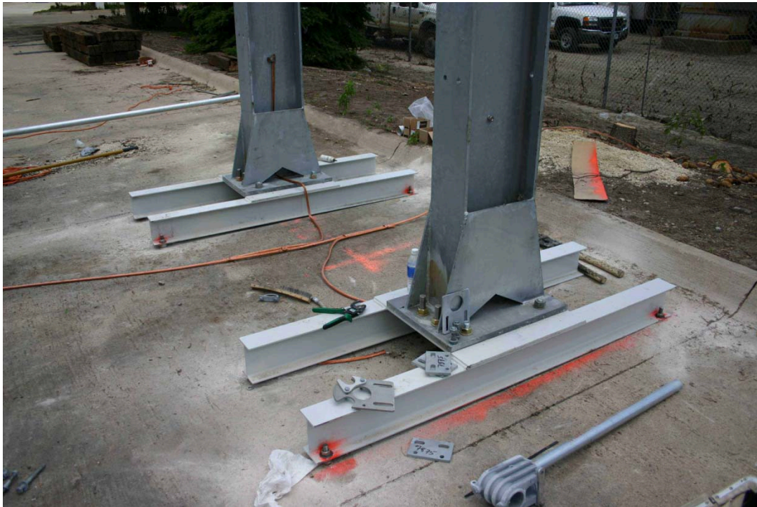
Figure – 4a Dead-End Tower Base
