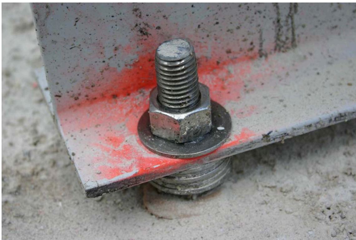
Figure – 4c Steel Base Secured With Epoxy Anchors
