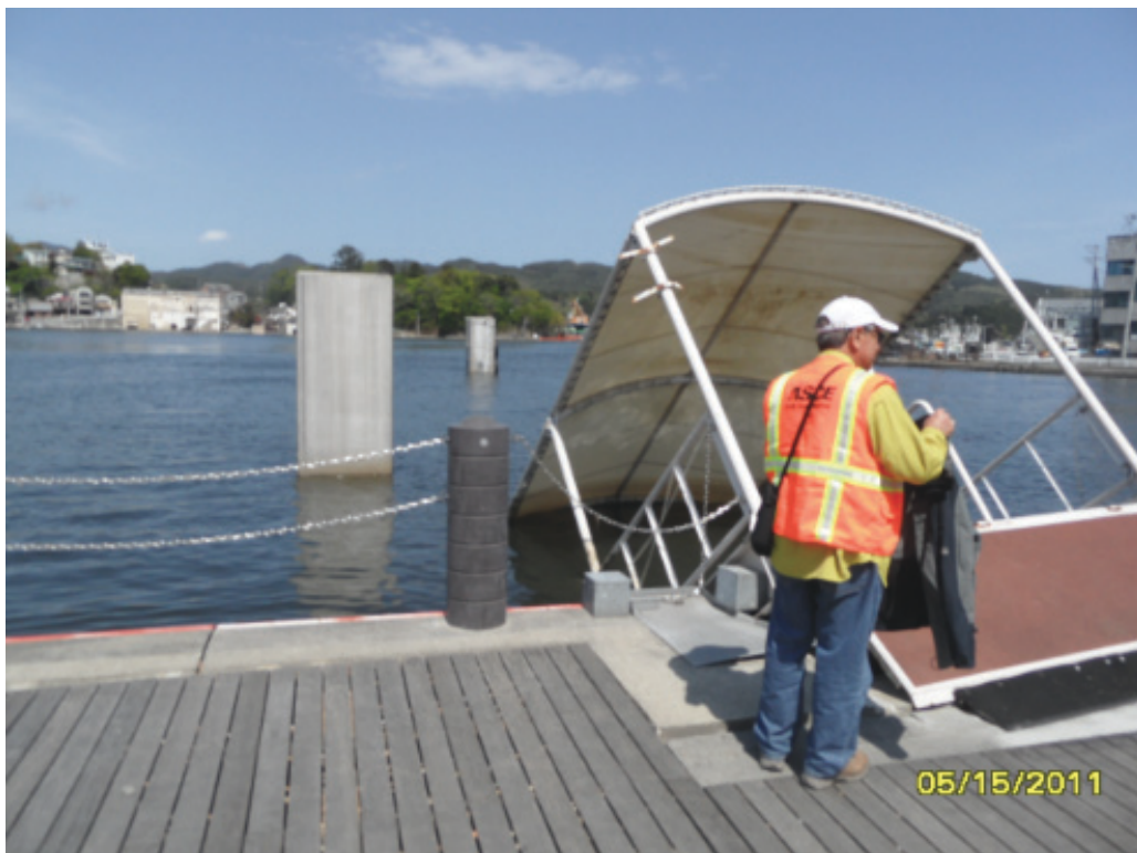
Figure 8-48 - Failed gangway and undamaged piles at Location 6 floating dock
