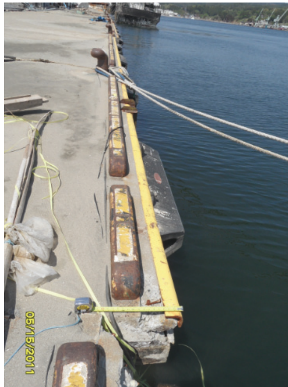
Figure 8-40 – Differential transverse movement of Location 5 wharf at construction joints
