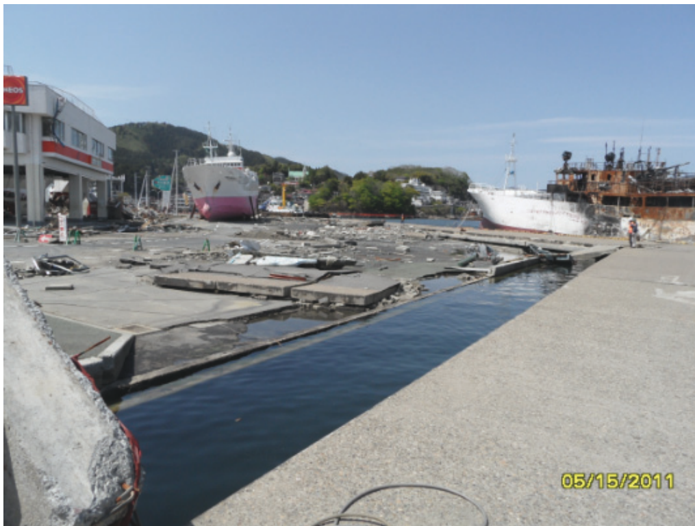
Figure 8-42 - Landside settlement at corner of Location 5 wharf
