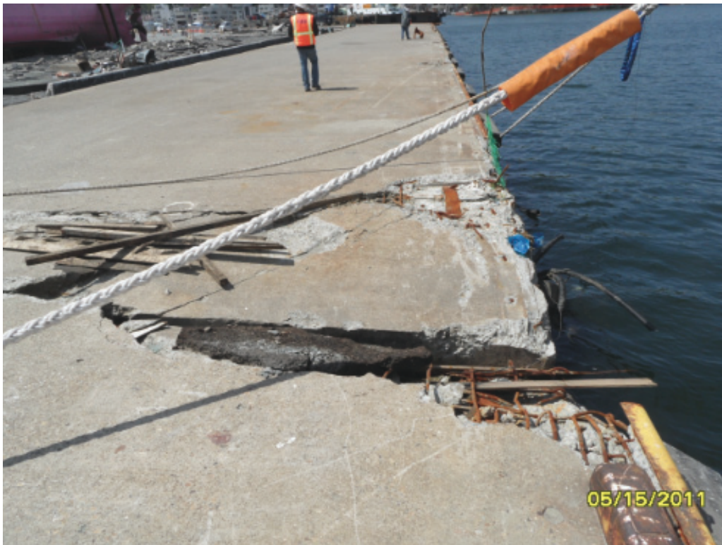
Figure 8-47 – Ruptured concrete anchorage for bollard at northern end of Location 5 wharf
