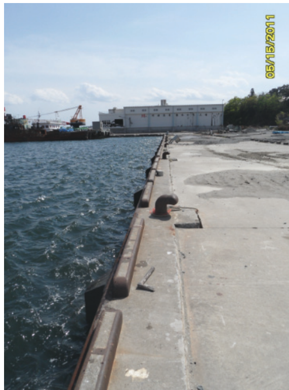
Figure 8-50 – Sheetpile wall wharf at Location 7 with limited settlement and no obvious movement
