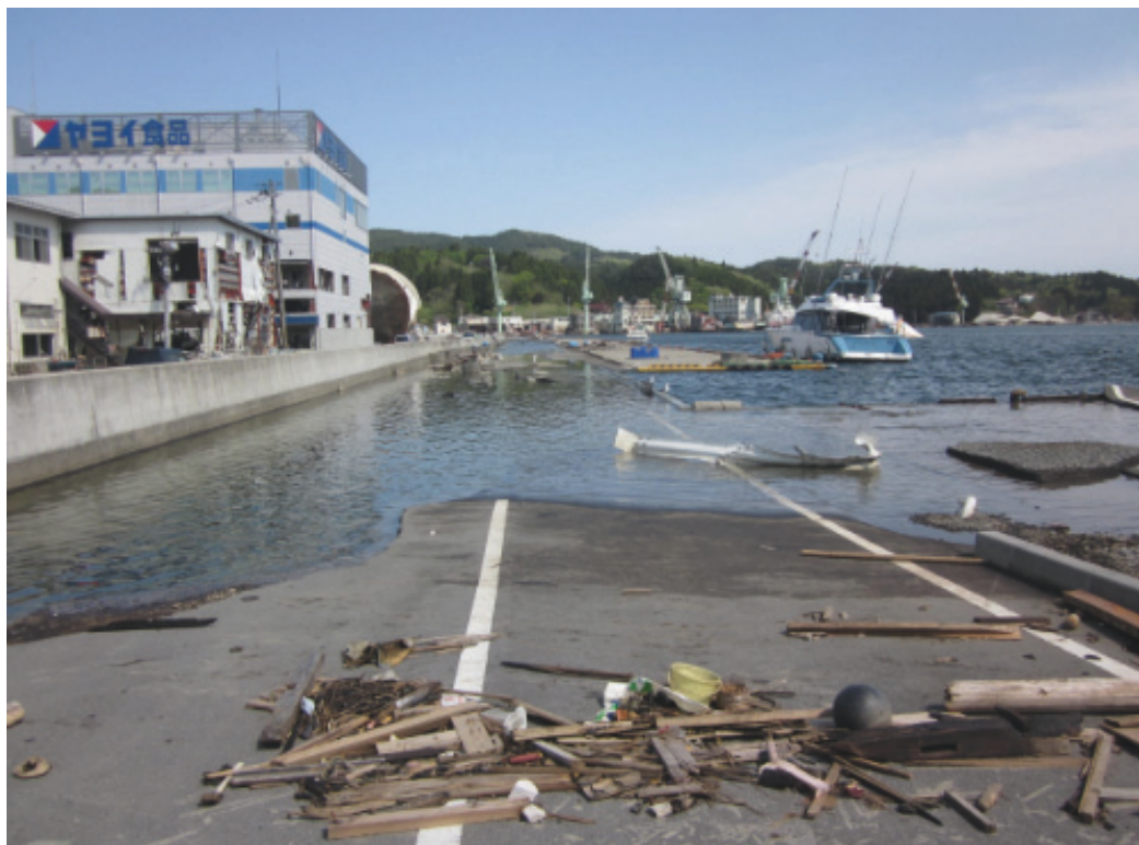
Figure 8-52 - Significant settlement behind gravity caisson wharf at Location 7
