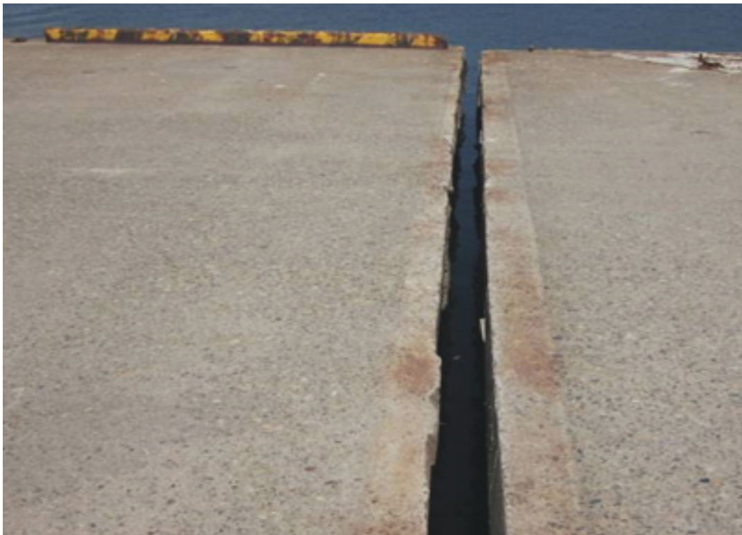
Figure 8-43 – Expansion joint separated 50 mm to 100 mm
