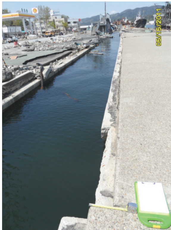
Figure 8-41 - Landside settlement along the wharf at Location 5 wharf
