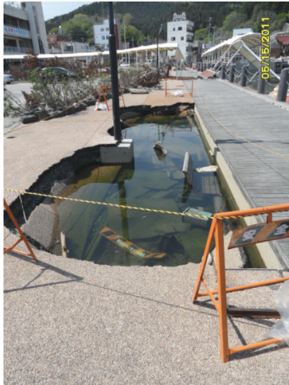
Figure 8-49 - Small area of Location 6 pedestrian wharf likely scoured away
