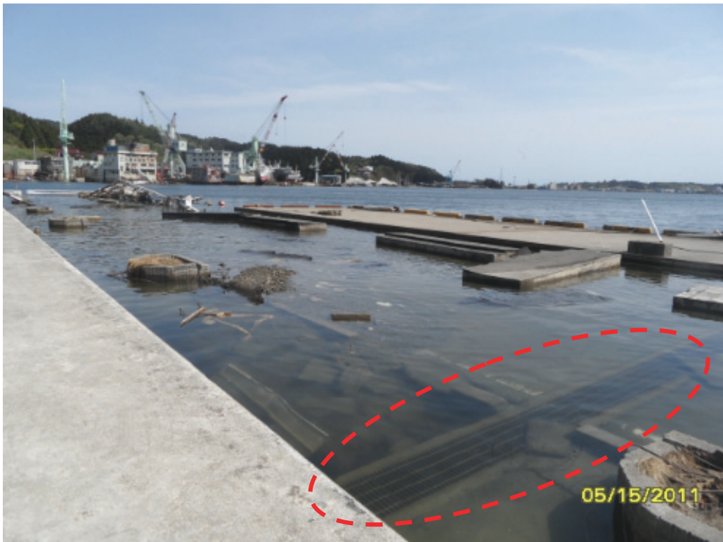
Figure 8-53 - Undamaged drainage grating and planters at backland settlement behind gravity caisson at Location 7
