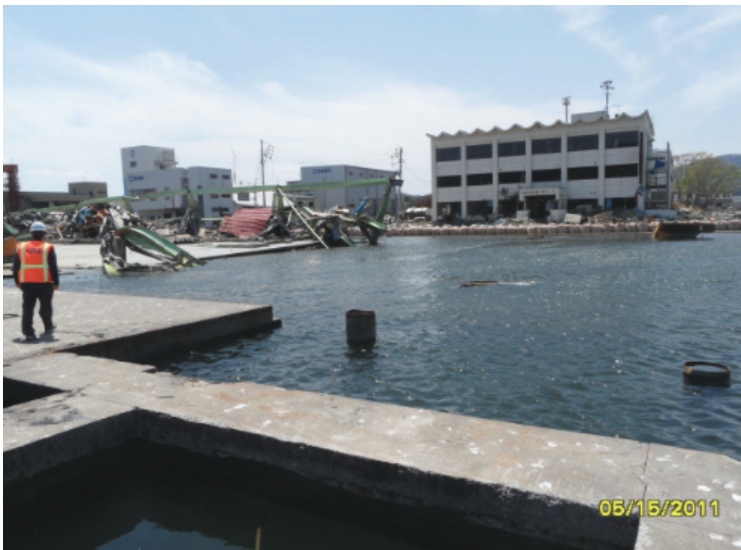
Figure 8-38 - Failed landside behind demolished wharf area
