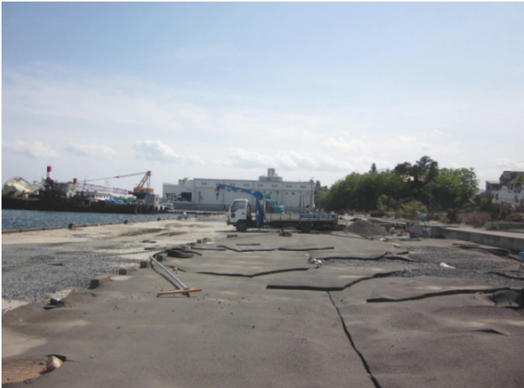
Figure 8-51 - Sheets of asphalt scoured from the deck surface at the Location 7 wharf
