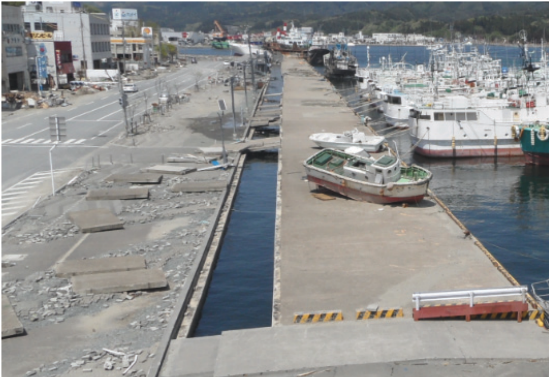
Figure 8-39 – Ramps popped out of place due to tsunami uplift loads
