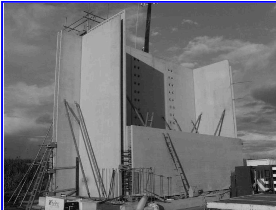
Figure 3 – Construction of ‘trial’ twinwall water-retaining tank at Laing O’Rourke’s manufacturing facility near Worksop
