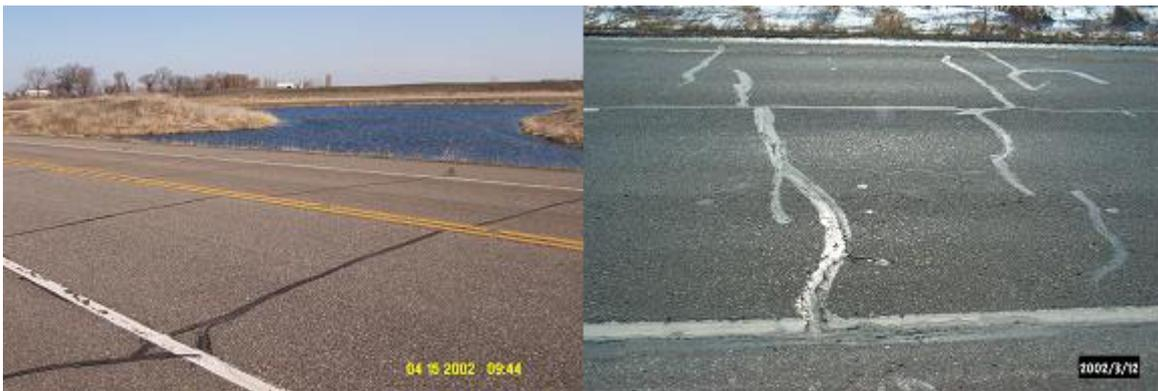
**Figure 4. Typical Cracking Patterns on PG 58-28 (left) and 64-22 (right) Cells**
