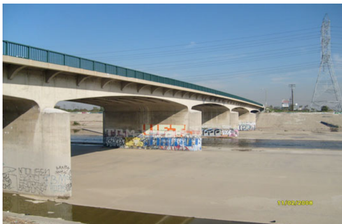
Figure 2. Sideview Gage Avenue Bridge Over L.A. River
