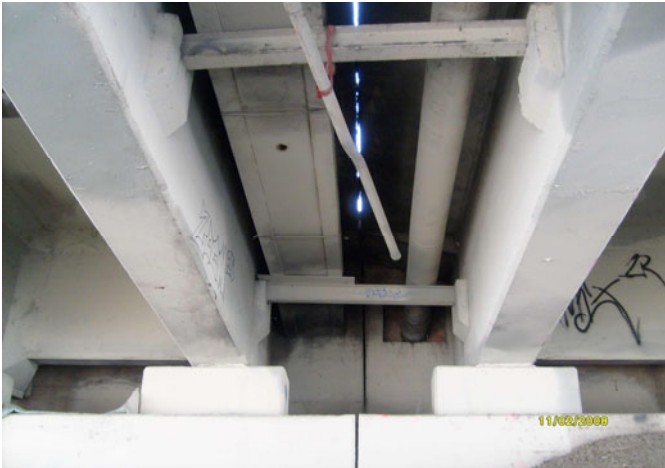
Figure 3. Existing Utilities Resting on Cross Beams
