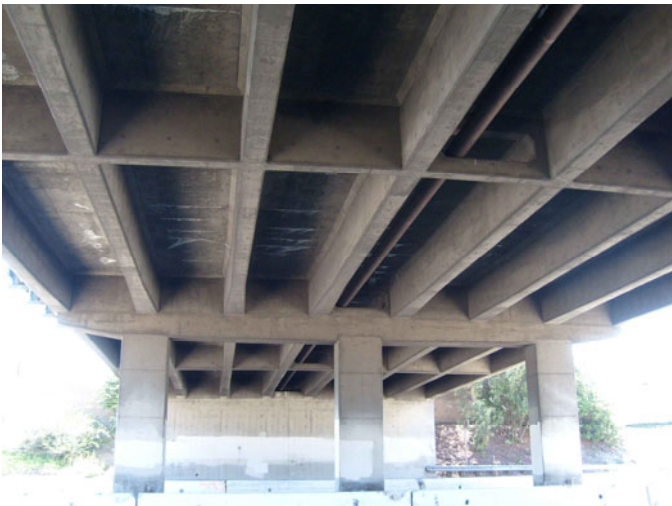
Figure 4. 710 Freeway Bridge Showing Blockouts for Utilities
