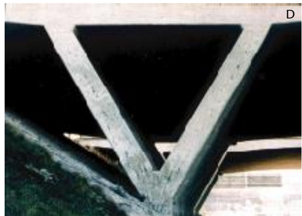
(d) Longitudinal cracking following the stress fields in reinforced concrete column of a 25-year-old highway bridge affected by AAR.
