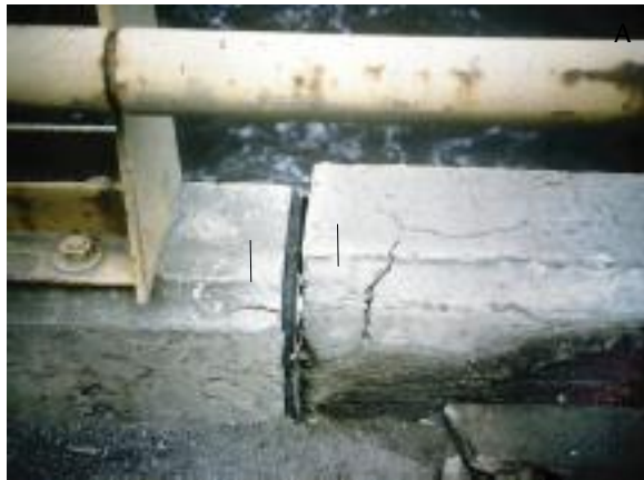
(a) Relative movements between pier blocks of a 15-year-old concrete dam affected by AAR; ASR cracking is also observed.
