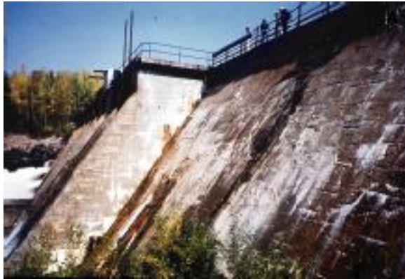
(a) Seepage of reservoir water along horizontal cracks and construction joints and associated leaching in a 50-year-old concrete dam affected by AAR.
