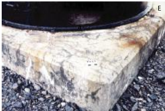
(e) Map-cracking (a) and associated leaching (b) in a 25-year-old transformer concrete foundation affected by AAR.
