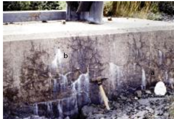
(f) Map-cracking (a) and gel exudation (b) in a 20-year-old electricity tower concrete foundation.
