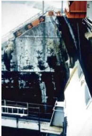
(e) Expansion and cracking due to AAR in a wing wall of the above structure, causing problems in operating the sluice-gate.
