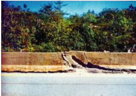
(a) Severe cracking and spalling of concrete due to AAR in a 20-year-old median highway barrier; freeze-thaw action has greatly influenced the extent of deterioration.
