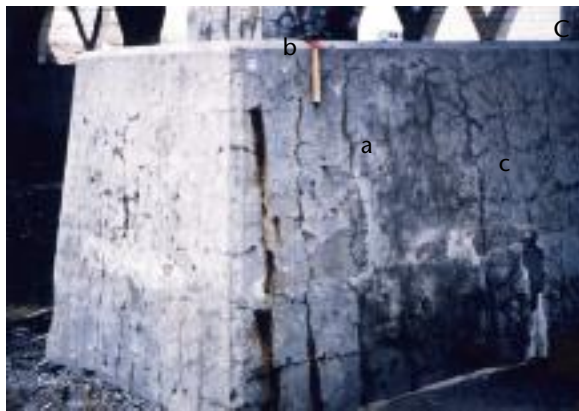
(c) Regular cracking pattern influenced by the presence of reinforcement in the massive concrete foundation of columns of a 25-year-old highway bridge affected by AAR (a). Cracking due to AAR accelerates deleterious processes such as corrosion of reinforcing bars (b). Gel exudations and efflorescence can also be observed (c).
