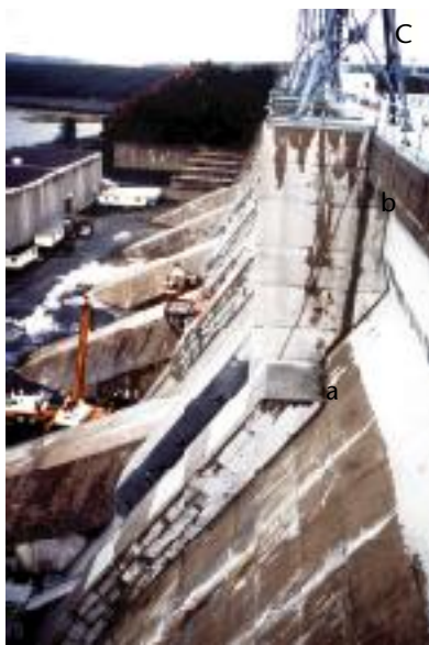
(c) Cracking on the downstream face (a) and in the upper part of a pier pedestal (b) of a 25-year-old dam affected by AAR.
