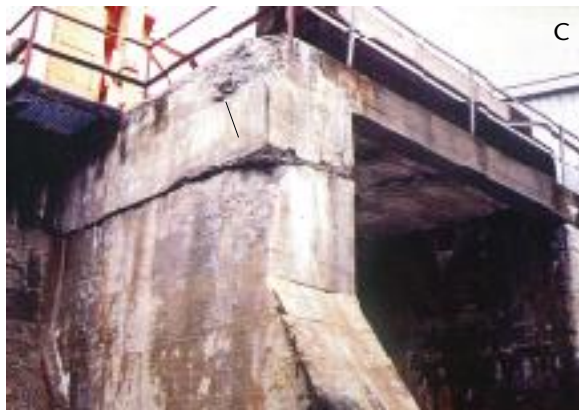
(c) Relative movement of a concrete pier caused by the expansive forces generated by the adjacent retaining wall (on the left).
