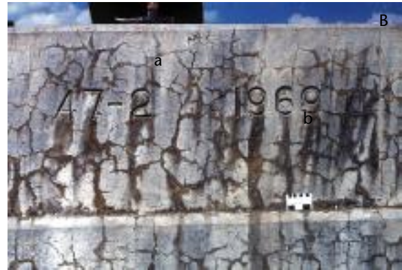
(b) Map-cracking due to AAR affecting the parapet wall of a 25-year-old highway bridge (a). Cracks show typical staining giving the appearance of permanent dampness (b).
