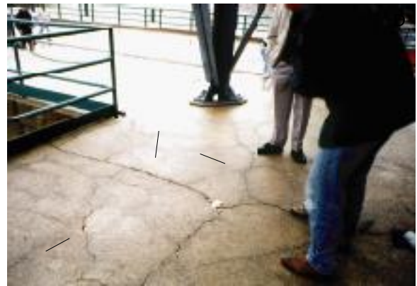
(d) Pattern-cracking on the top of a pier block of the dam shown in Figure 5(c).
