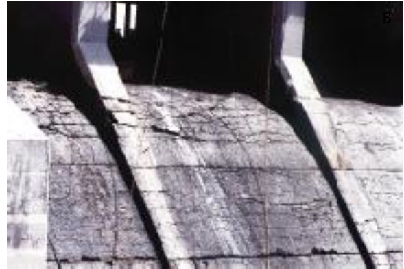
(b) Severe horizontal cracking in the spillway of a 15-year-old concrete dam affected by AAR.
