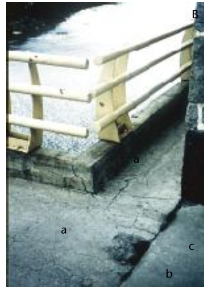
(b) Relative movement between a pier block shows cracks due to ASR (a) and the adjacent deck slab of the above dam causing spalling of concrete (b) and extrusion of sealing material along the joint (c).
