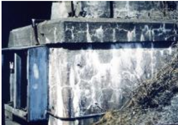
(e) Exudations of alkali-silica gel at the surface of a concrete foundation adjacent to a 25-year-old highway bridge.
