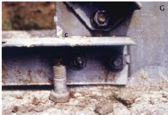
(g) Expansion of the concrete has caused shearing of steel bolts (c).
