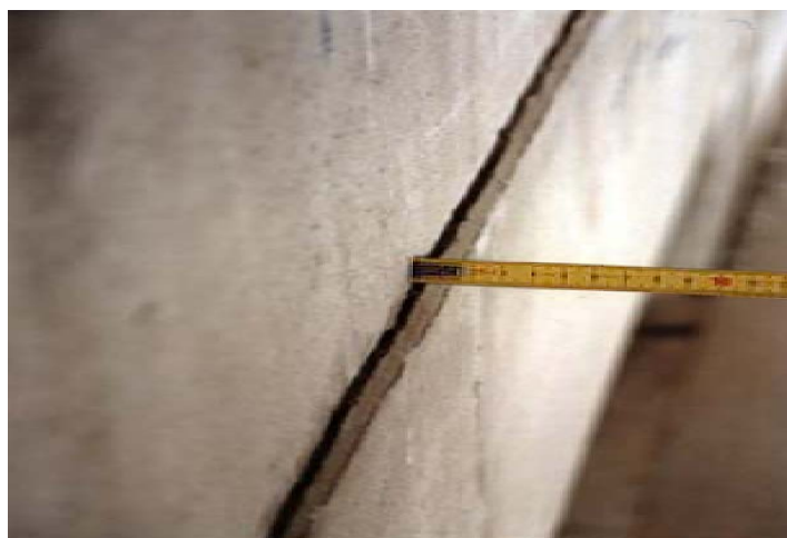
Figure 2: 15 mm (0.6 in) displacement of the limestone facing block caused by beam corrosion.
